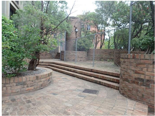
Figure 32 –common area exterior.
