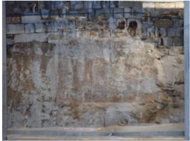
Figure 30 – sandstone bedrock cut for the boiler room basement, with sandstone blocks present on top of the bedrock.
