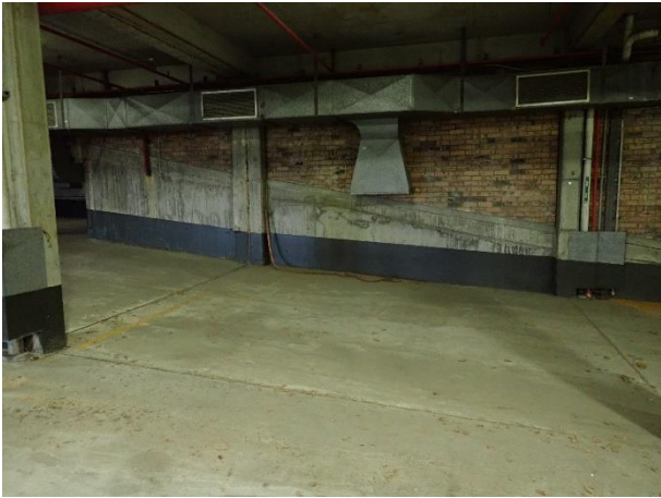
Figure 29 – basement parking level with brick wall.
