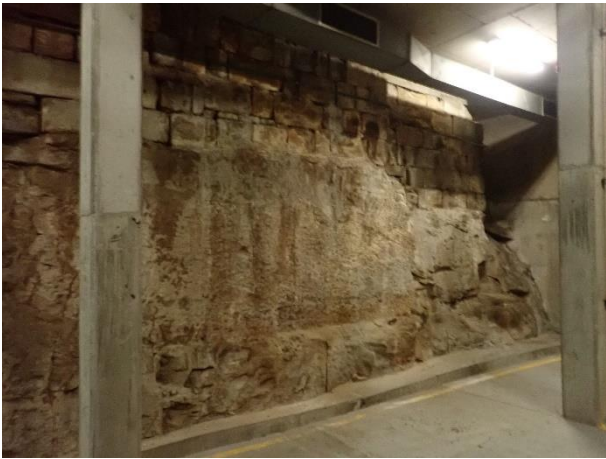
Figure 31 – sandstone bedrock cut for the boiler room basement, with sandstone blocks present on top of the bedrock.
