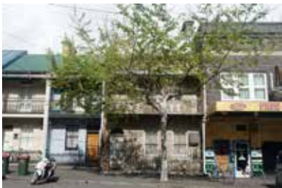
Figure 02: 128 Regent Street Terrace
