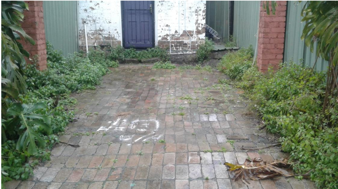
Photograph 6: Rear of No. 94 Regent Street
