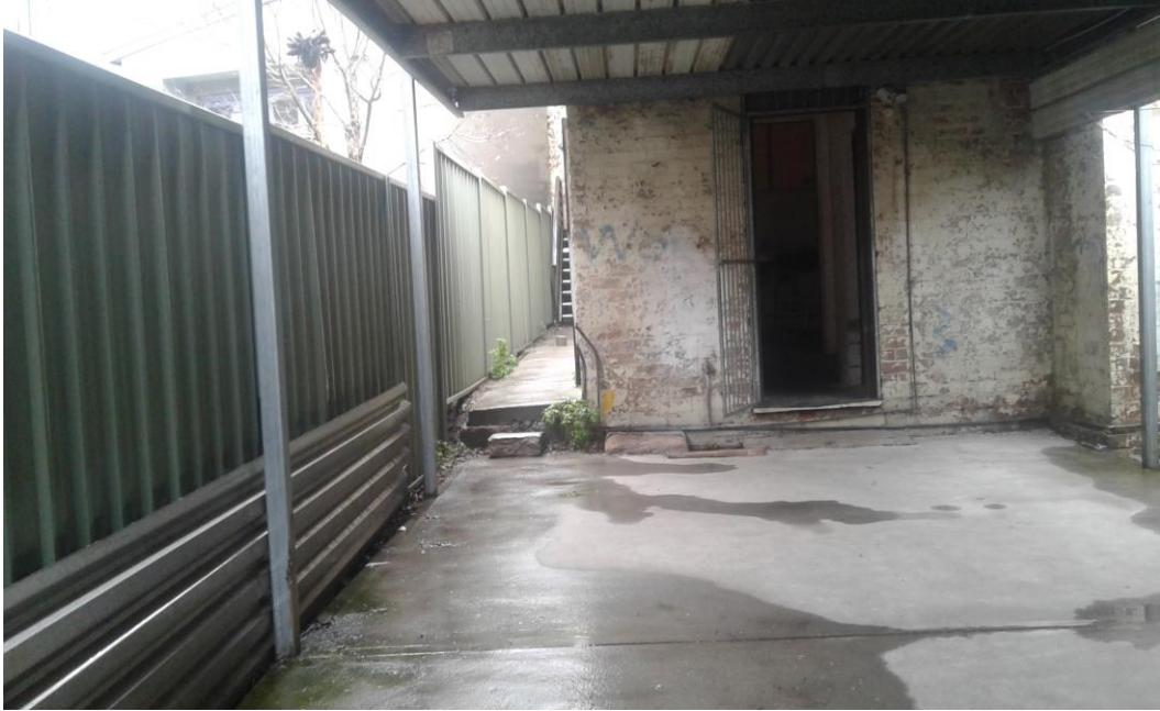
Photograph 3: Rear of No. 92 Regent Street
