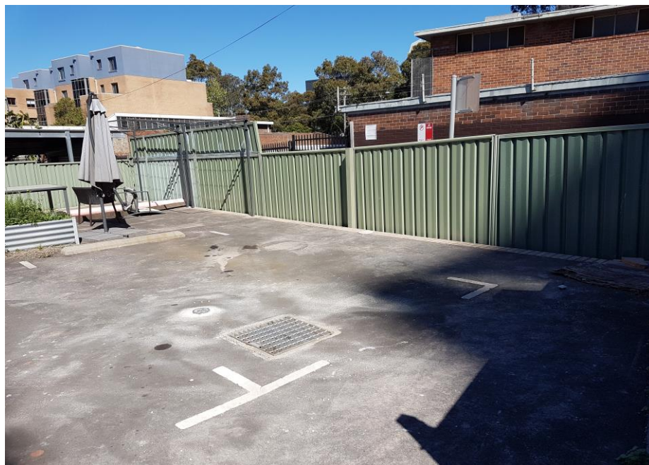
Photograph 2: Rear of No. 90 Regent Street
