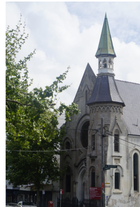
Figure 01: View of 'St Lukes Presbyterian Church'
