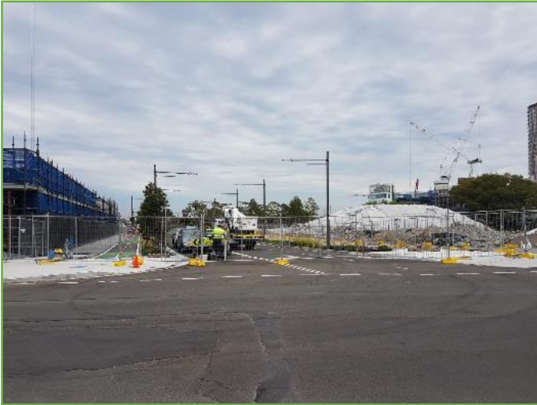
View looking west at intersection of Geddes Avenue and Portman Street
