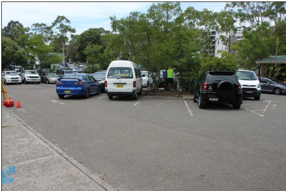
Figure 5-14 Asphalt carpark on the study site, facing north east. AMAC Group IMG_2173, (22/01/2018).
