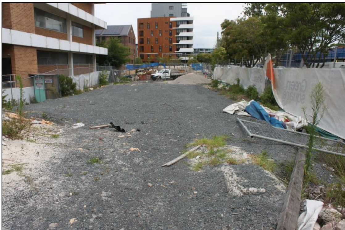
Figure 5-10 Western extent of the study site, note the gravel bedding/levelling fills, facing south. AMAC Group IMG_2153, (22/01/2018).
