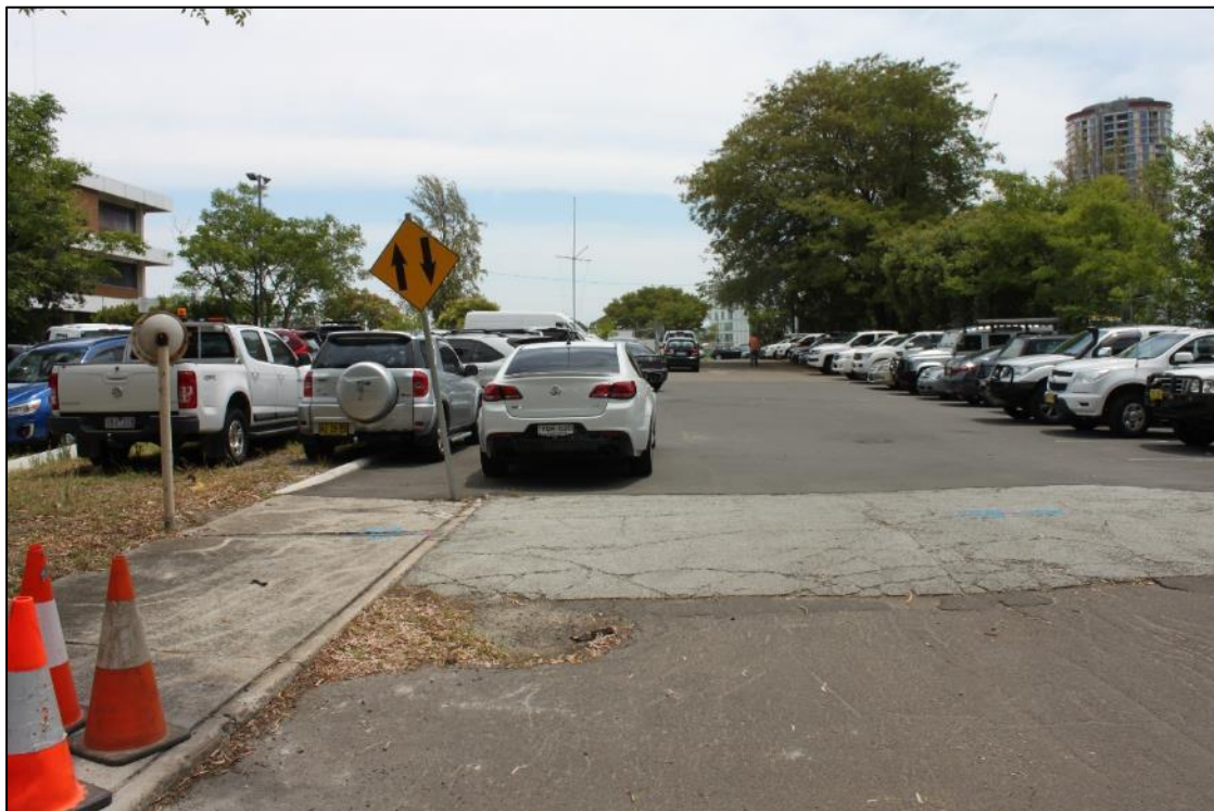
Figure 5-16 Asphalt carpark and driving fronting Joynton Avenue, facing west. AMAC Group IMG_2182, (22/01/2018).
