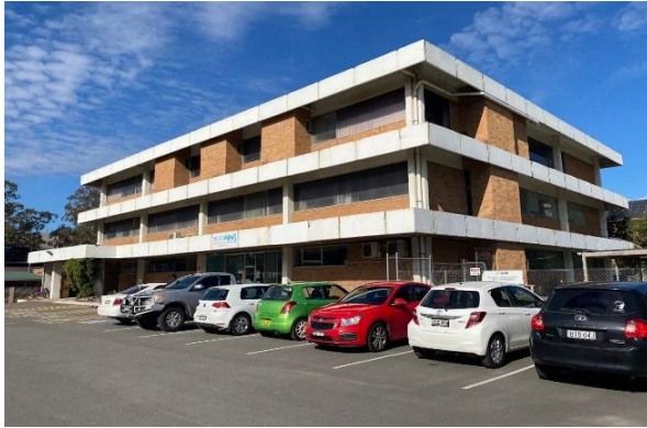
Figure 13: Exterior of the Hydrotherapy Building from northern carpark, view looking southeast (CPH, 26 June 2020).
