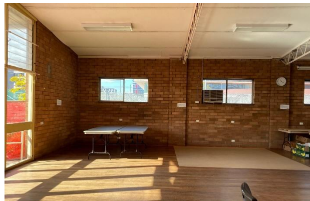
Figure 22: Interior of the Community Hall building, looking east (CPH, 26 June 2020).
