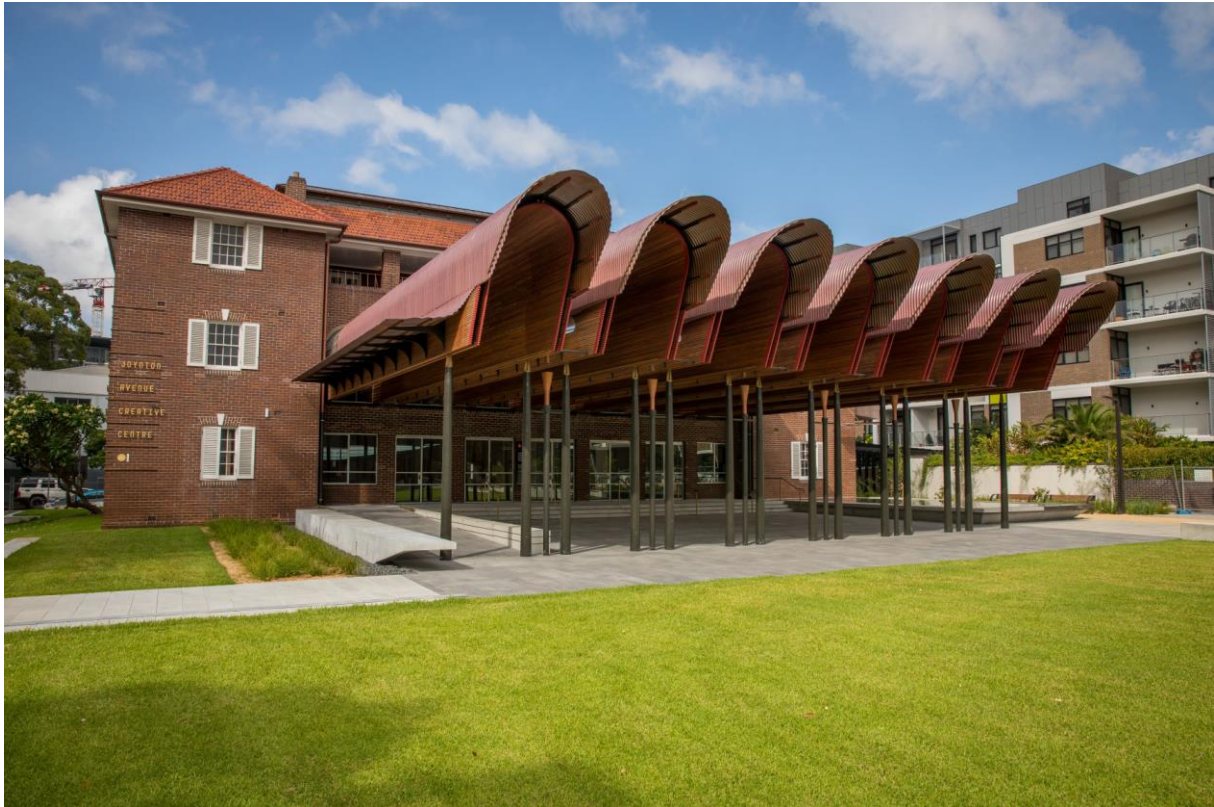
Figure 2: The Joynton Avenue Creative Centre which adaptively reused the former Esme Cahill Building (Source: https://news.cityofsydney.nsw.gov.au/articles/old-hospital-building-reinvented-as-award-winning-creative-hub )
