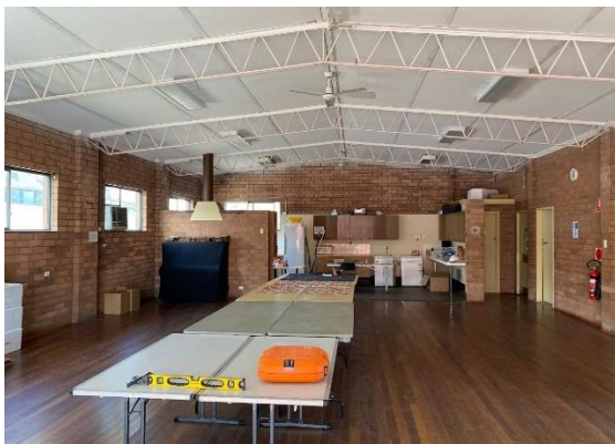
Figure 21: Interior of the Community Hall Building, looking south (CPH, 26 June 2020).
