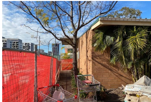
Figure 20: Northwest corner of the Community Hall building, showing utilitarian facebrick finish, view looking east (CPH, 26 June 2020).
