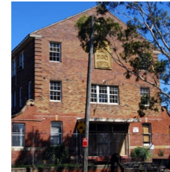
2. GREEN INFRASTRUCTURE CENTRE
