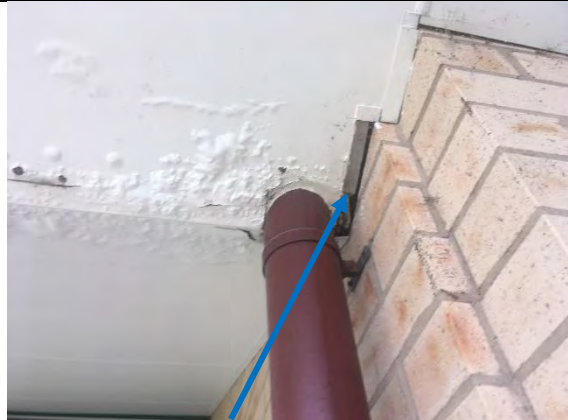
Photo 4 Eave linings - Villaboard No asbestos detected Sample No: E73071
