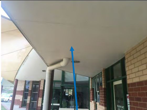
Photo 3 Eave linings - Villaboard No asbestos detected Sample No: E73071
