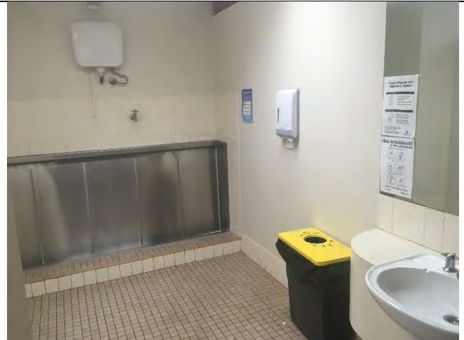
Photo 14 Internal wet areas No asbestos observed
