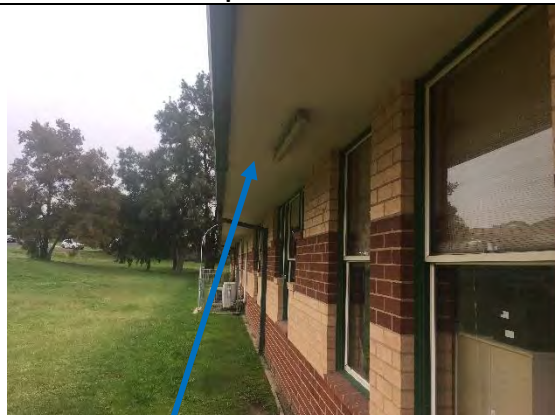
Photo 6 Eave linings - Villaboard No asbestos detected Sample No: E73071
