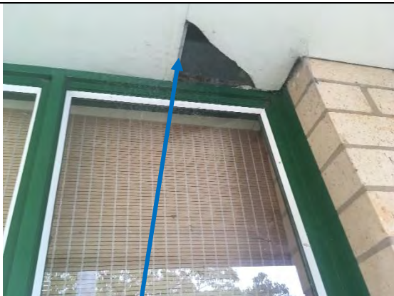
Photo 5 Eave linings - Villaboard No asbestos detected Sample No: E73071
