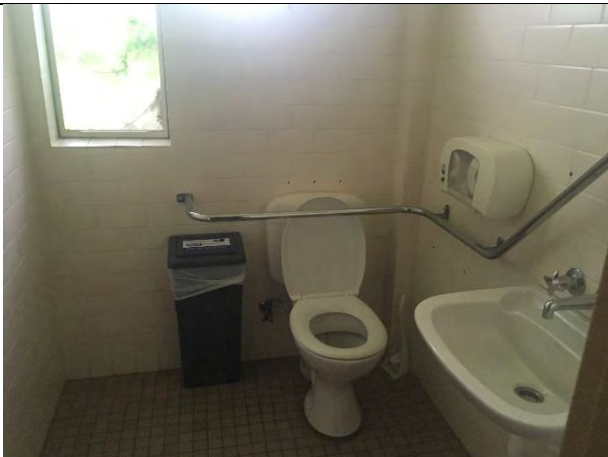
Photo 11 Internal wet areas No asbestos observed
