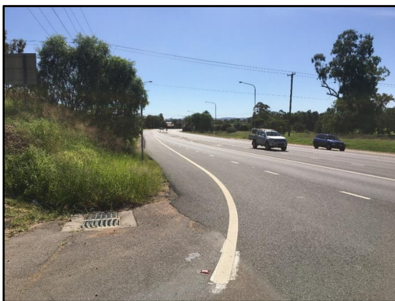
Photo 1 - View looking west (left out) along the New England Highway from existing driveway crossover.
