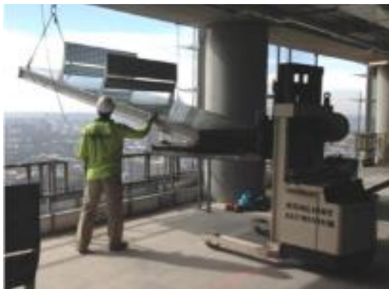
Figure 25 – façade Installation with a Walkie Reach
