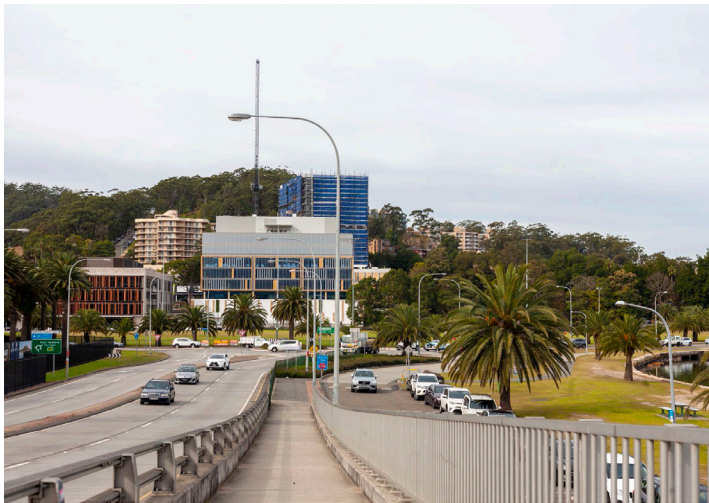
C. Brian McGowan Bridge
