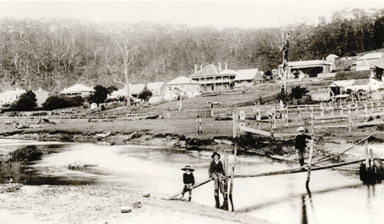
Mann Street Gosford from the creek now under Baker Street circa 1885, credit “Gostalgia” local history from Gosford Library
