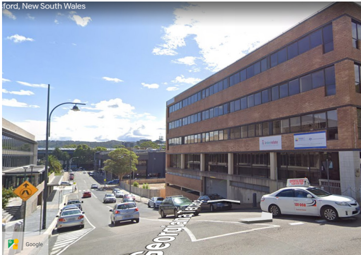
E. Mann St and Georgiana Tce intersection
