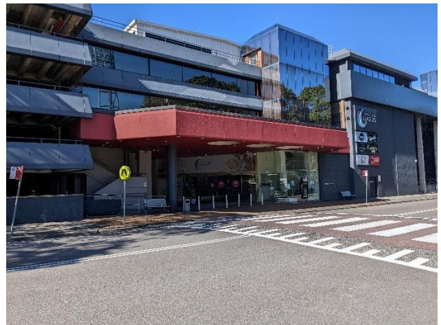
Picture 2 Main pedestrian entrance on Dane Drive
