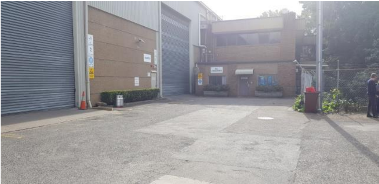
PHOTO 1 - In northern carpark looking west towards Office Building showing building downpipes
