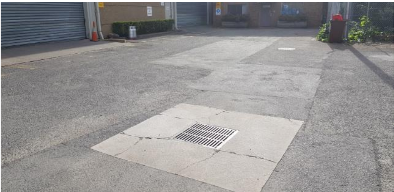
PHOTO 2 - Existing grated drainage pits in Northern Carpark
