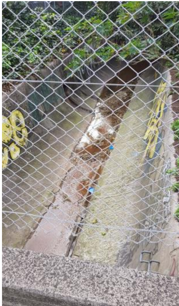
PHOTO 4 – Stormwater Drainage Canal looking west
