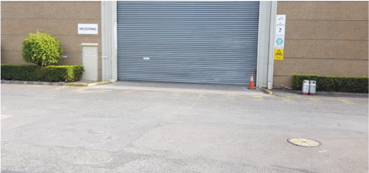
PHOTO 3 – Looking South at side entry roller door and downpipes
