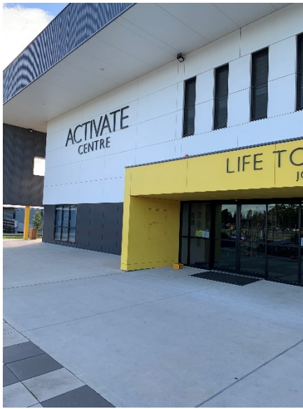
27. Looking southeast towards Building H1 (sports hall). No hazardous materials within exterior.
