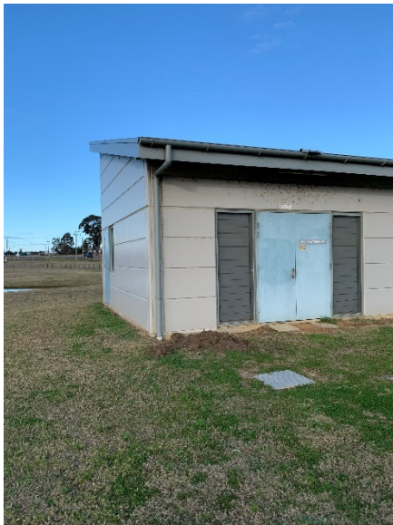
29. Looking west towards Building K (switch building / proposed café). No hazardous materials within exterior.
