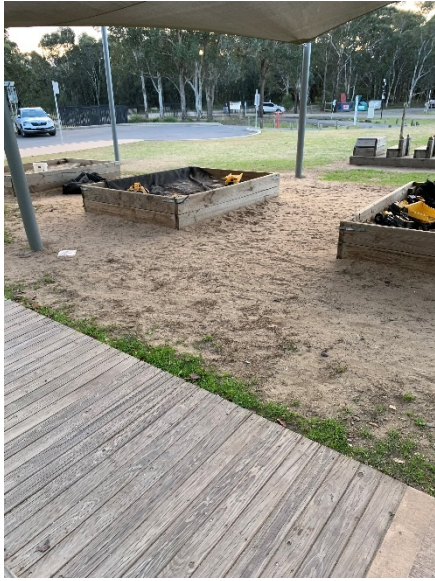
31. Looking northeast across Areas A3 and A4 (proposed extensions to building A1 No hazardous materials within exterior.
