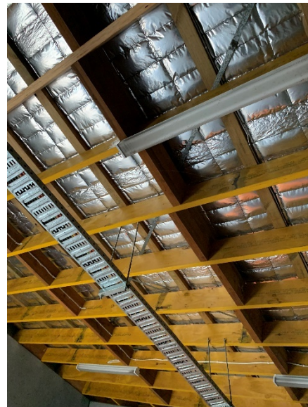
30. Looking northeast within Building K (switch building / proposed café). No hazardous materials within interior. Note that there is no insulation underneath the ceiling 'sarking', therefore no SMF.
