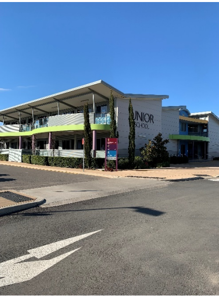
21. Looking southeast towards Building A1 (junior school). No hazardous materials within exterior.
