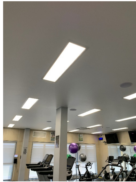
28. Sports Hall (H1 building) lower floor room (gymnasium) ceiling; SMF understood to be present within cavity based on discussion with maintenance personnel
