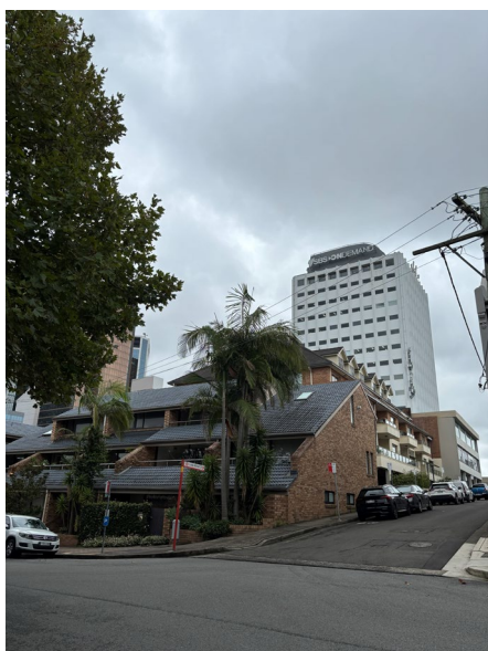
263 Alfred Street, looking north
