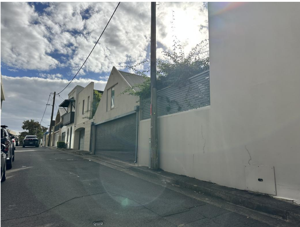
Figure 22 View to the Whaling Road Conservation Area from Little Alfred Street looking north-east
