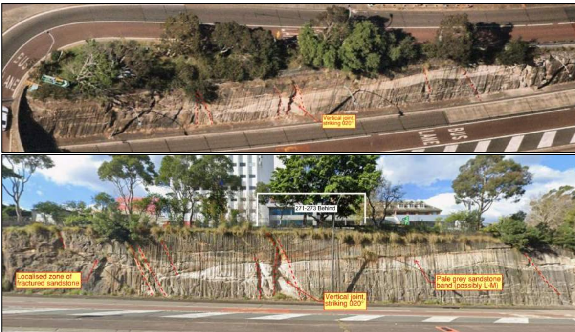
Figure 3: Ortho photograph dated 5 May 2018 (above) and Google Maps Street View dated June 2021 (below) showing rock face prior to Warringah Freeway works, and marked up joints (red). Both photographs looking east.
