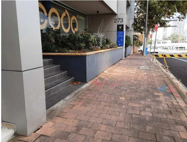
Photo 15 Street view showing the multi-storey building facing Alfred Street [10] extant where dwelling [8] was located, facing south-east
