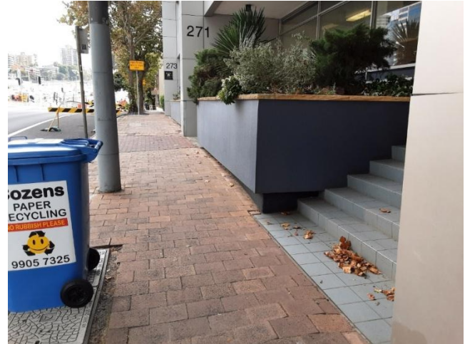
Photo 16 Street view showing the multi-storey building facing Alfred Street [10] extant where dwelling [8] was located, facing north
