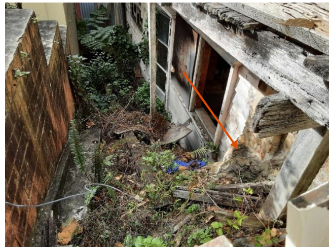
Photo 22 View of house on eastern site of Little Alfred Street with a brick pier built atop a natural stone outcropping, facing east
