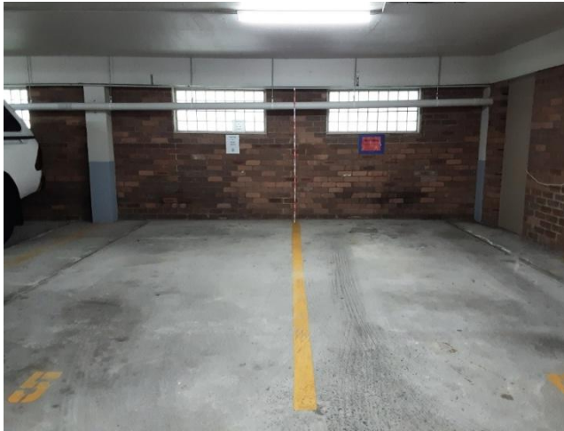
Photo 19 View of the basement associated with [10] showing the windows at street level, facing west
