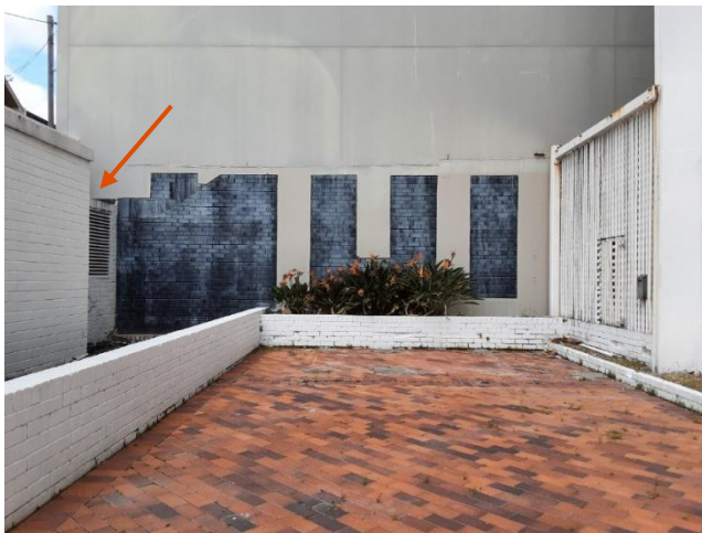
Photo 17 View indicating the street level (orange arrow) above the floor level of the building facing Little Alfred Street [11], facing south
