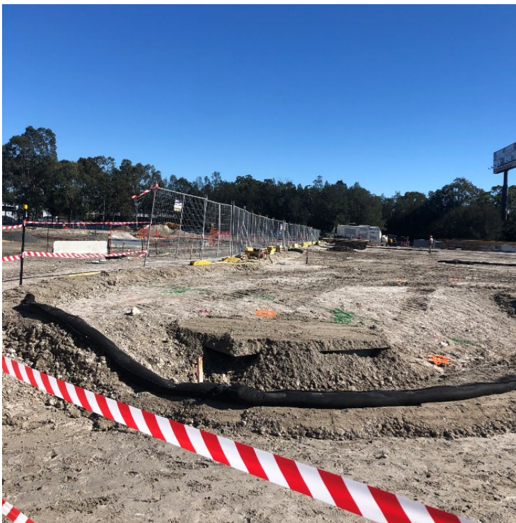
First Piling site hole prepared
