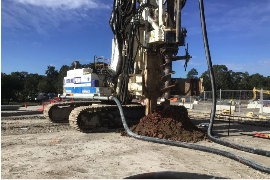
First piling hole
