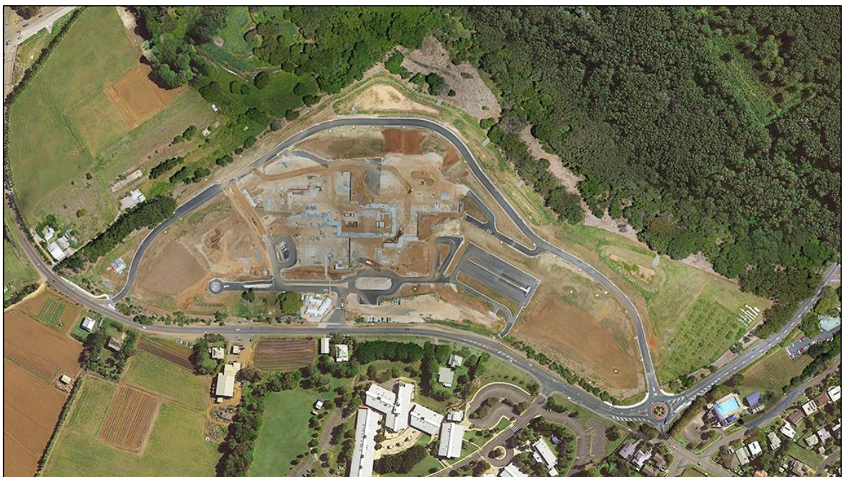
Plate 2.1 Tweed Valley Hospital Site, November 2020
