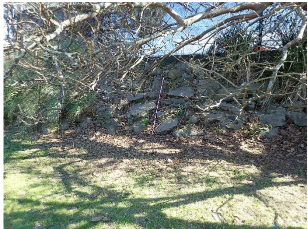
Figure 18 – Retaining wall on eastern perimeter of subject area/school boundary, facing W.
