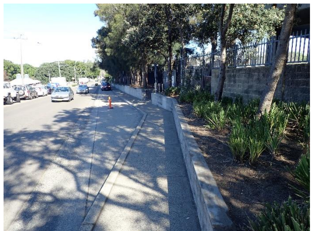
Figure 20 – Concrete retaining wall along north-western perimeter of school, facing S.
