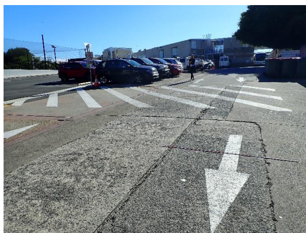
Figure 14 – Carpark in the south section of the subject area, north of York Rd, facing N.
