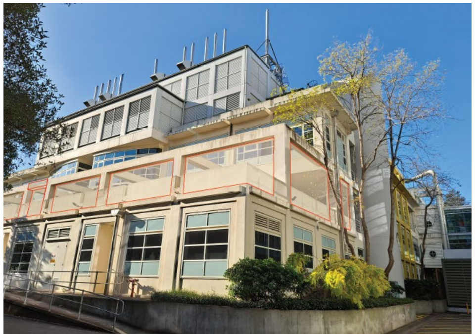
Figure 5 Infill of existing masonry (infill location shown in red) as part of the Pathology refurbishment.
