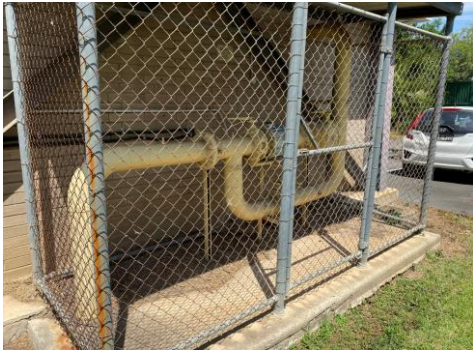
Figure 5 - Gas line to CHW site
