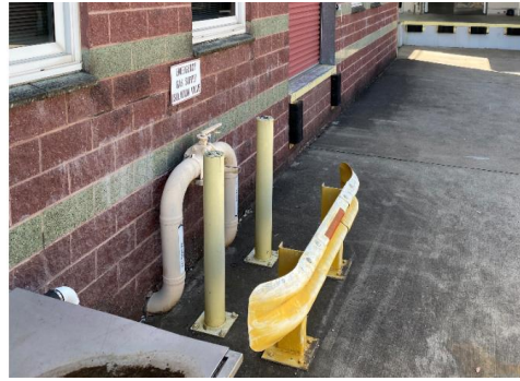
Figure 6- Isolation valve in loading dock
