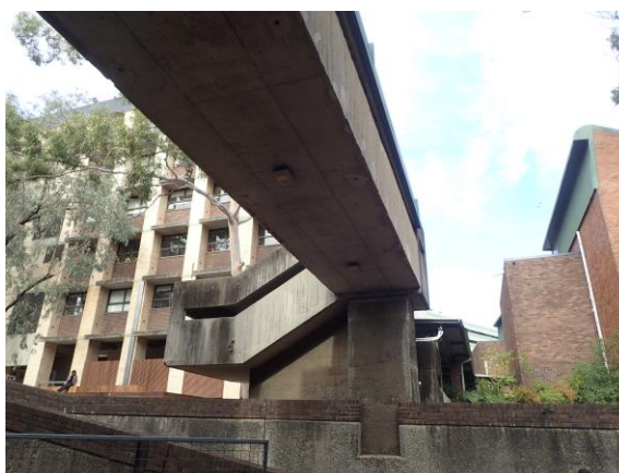
Figure 5.23 Detail of the concrete bridge. Note the concrete formed roof of the stairs, also note the visible formwork as is typical of brutalist architecture.
