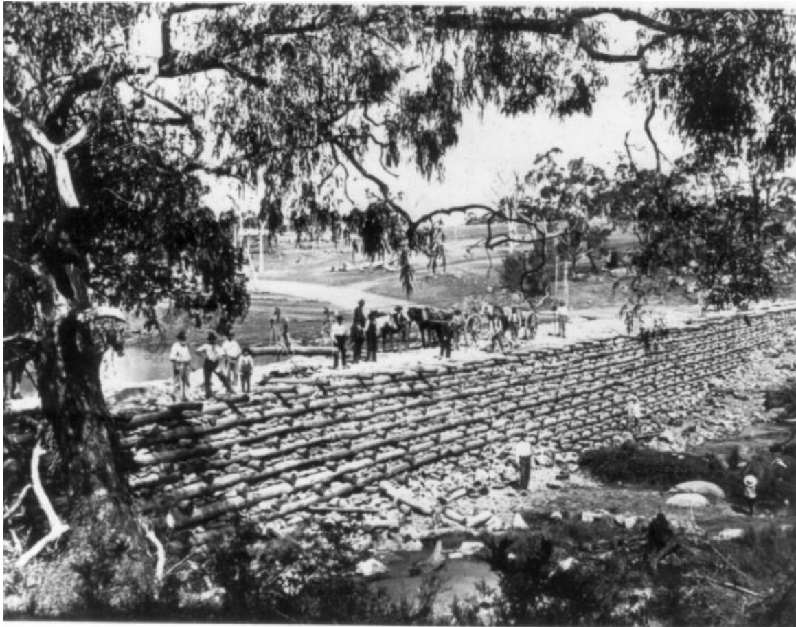
Figure 3-5 Dam under construction across the Gara River at Blue Hole under construction c. 1899-1900 (Gojak 1988:5).
