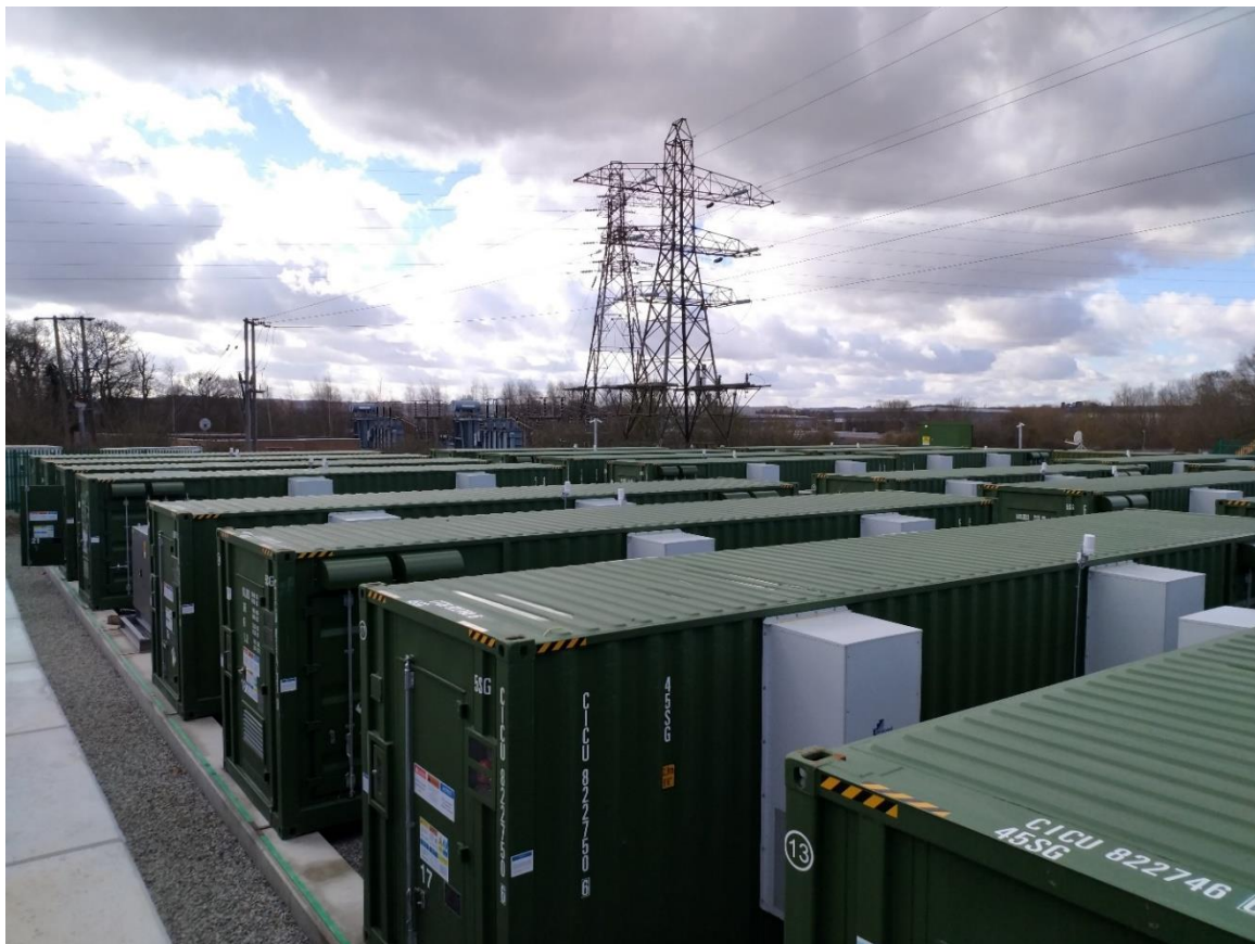
Figure 1-12 Typical battery storage units, located together.
