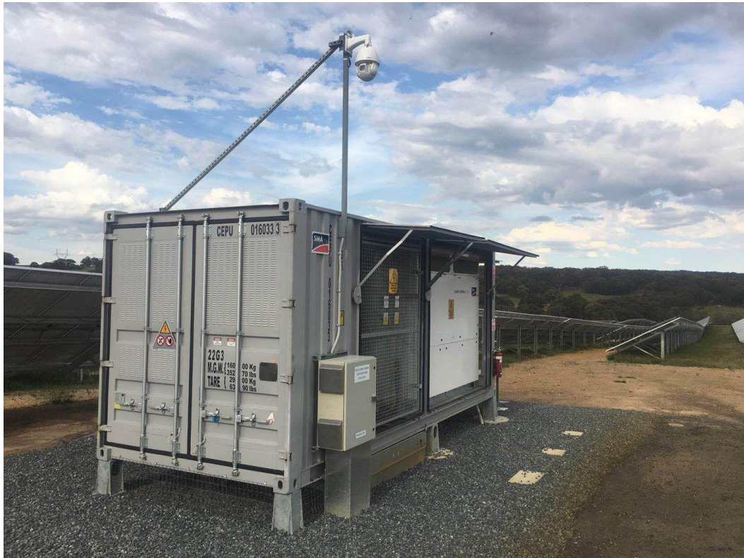
Figure 1-8 Typical illustration of a PCU within the array.
