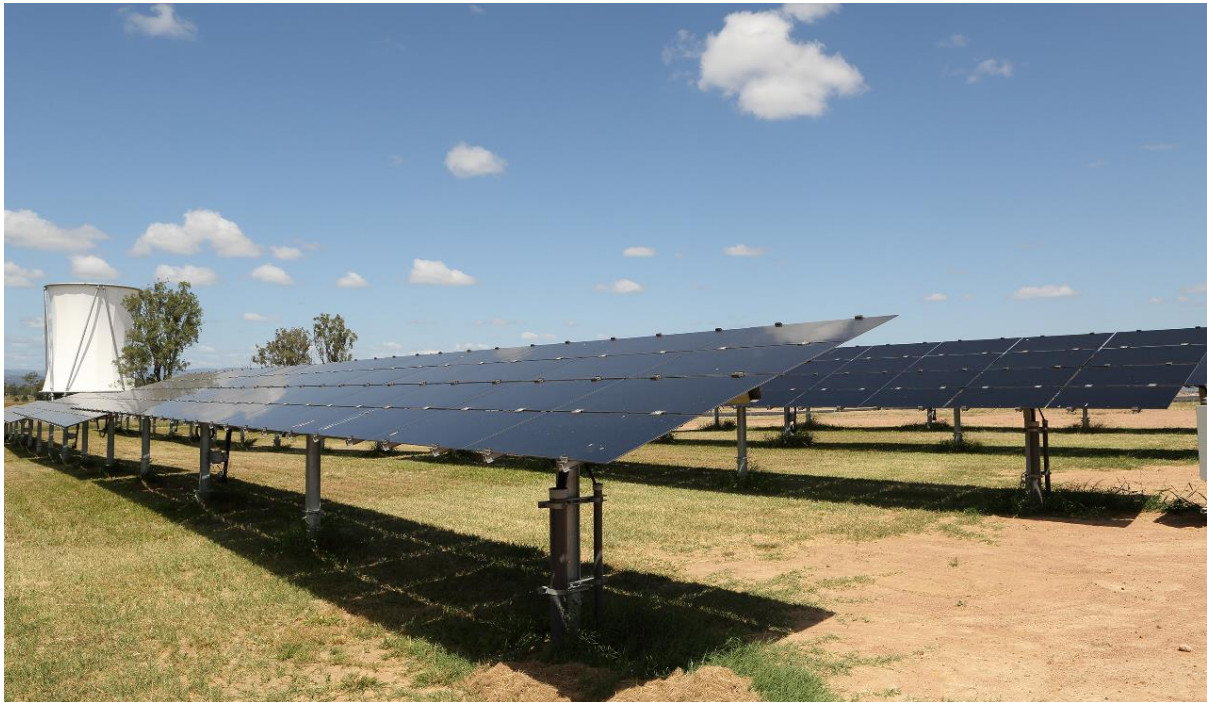
Figure 1-6 Typical single-axis tracking system.
