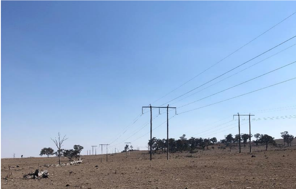
Figure 1-9 Existing 132kV transmission lines traversing the proposal site that will connect the solar farm to the Armidale substation.
