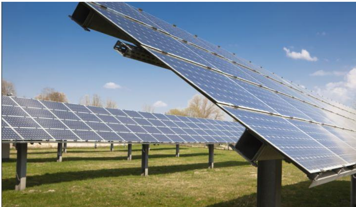
Figure 1-5 Typical fixed tilted system.
