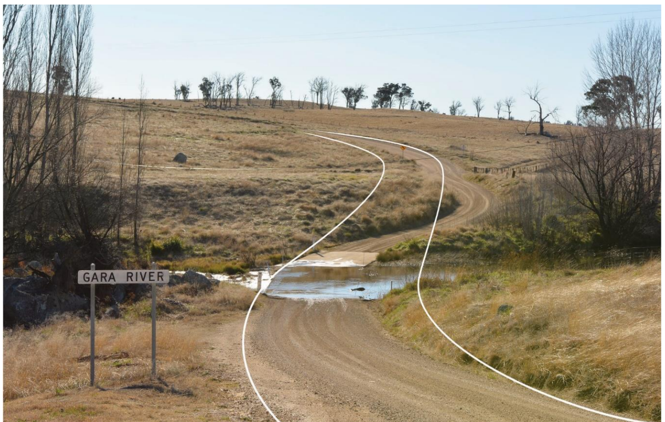
Figure 1-10 Concept of Causeway Upgrading, Gara Road Chainage 9.05km
