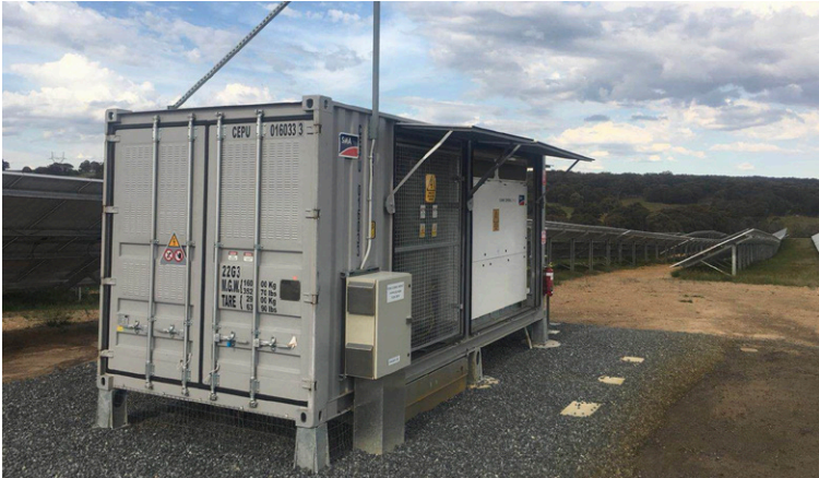
Image 04. Typical Power Conversion Unit (PCU) (Source: NGH)
