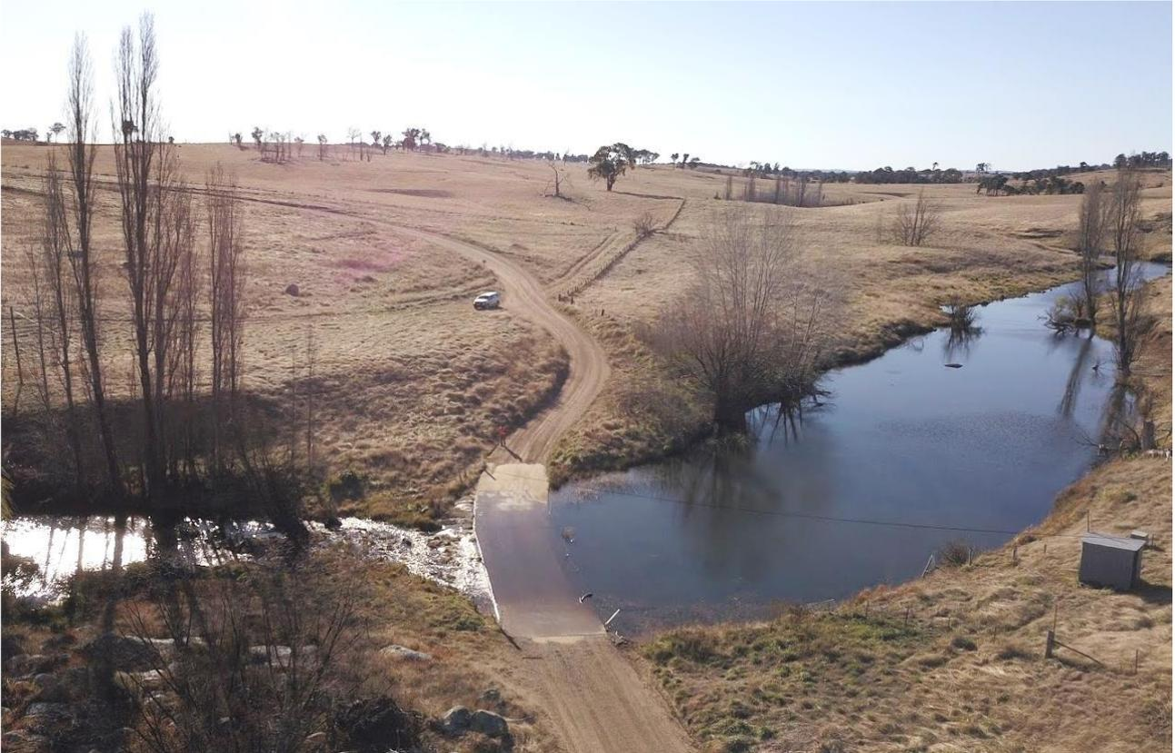
Figure 8-15 Causeway Crossing of Gara River on Gara Road, Chainage 9.05km.
