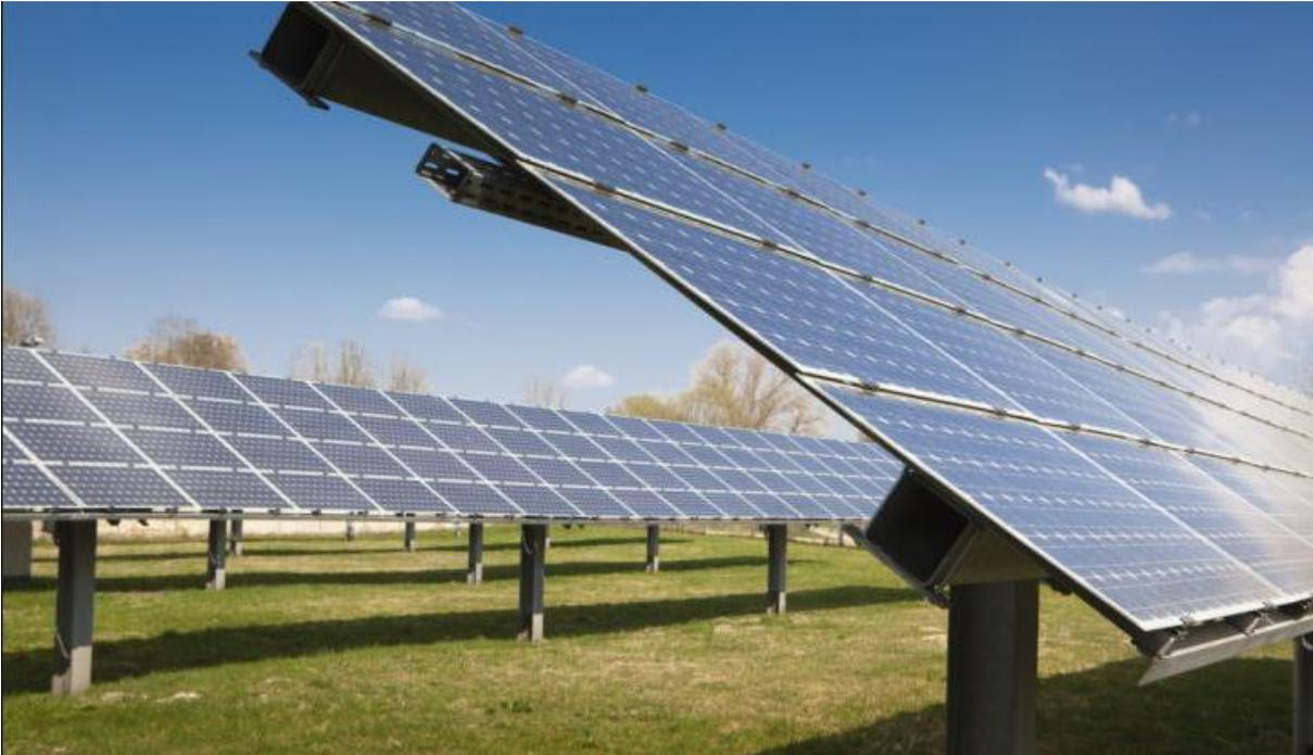
Figure 4-2 Typical fixed tilted system.
