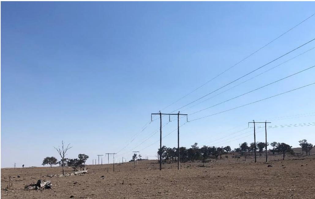
Figure 4-6 Existing 132kV transmission lines traversing the proposal site that will connect the solar farm to the Armidale substation.
