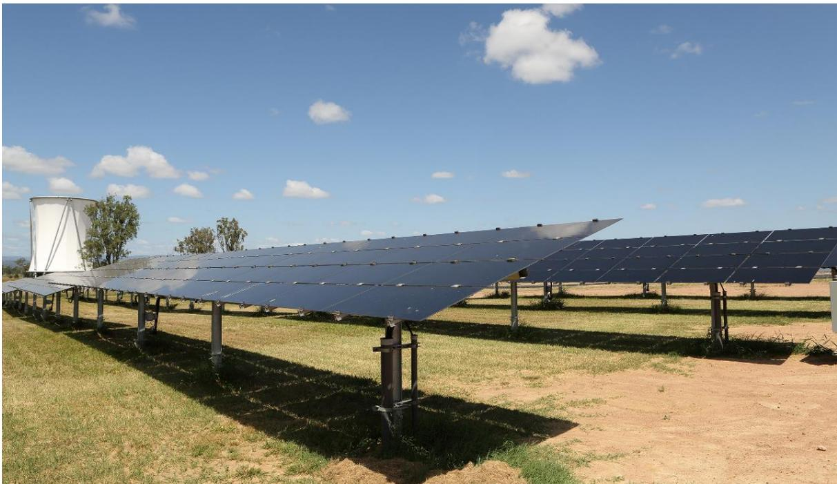
Figure 4-3 Typical single-axis tracking system.
