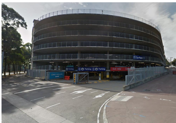
Figure 5 P1 carpark, as viewed from Edwin Flack Avenue
