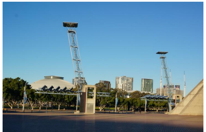
Figure 10 Buildings above the tree line to the east of Olympic Boulevard
