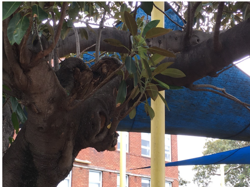
Figure 2 - Decay at Location 1
