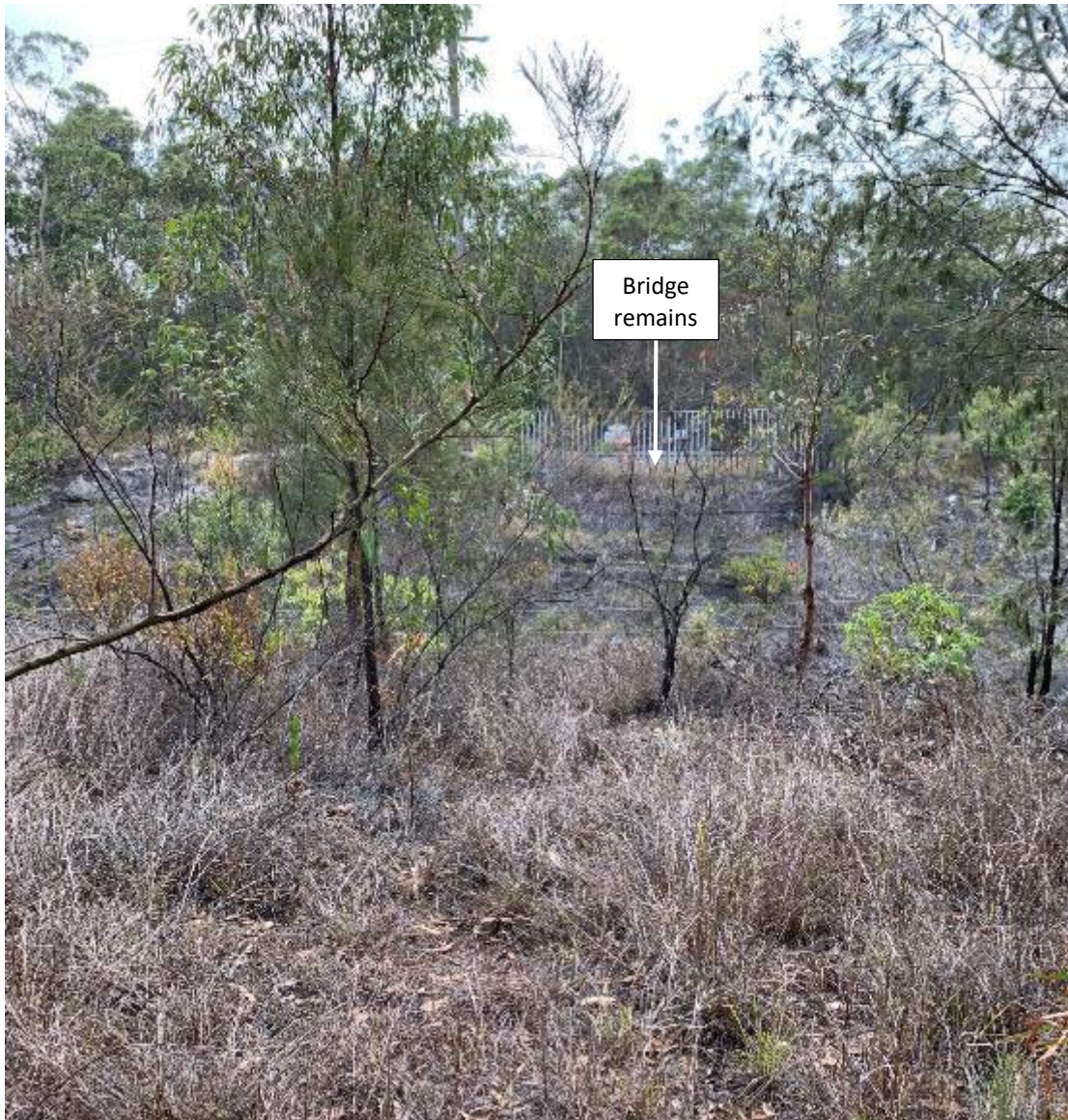
Plate 5.24 View of the Bridge remains facing west over the Great Northern Railway
