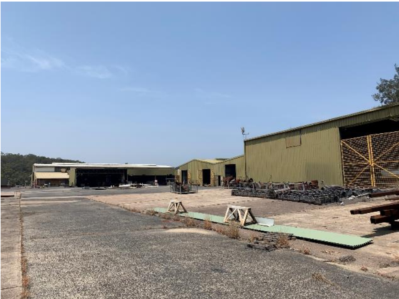
Plate 5.5 Views within Newstan Colliery, showing post-1948 building stock
