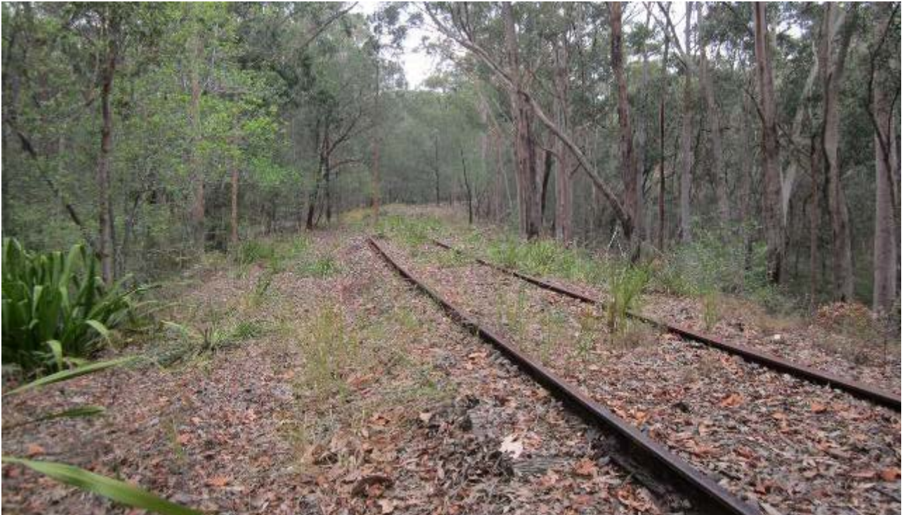
Plate 5.16 View of a section of the Line that extends along an embankment
