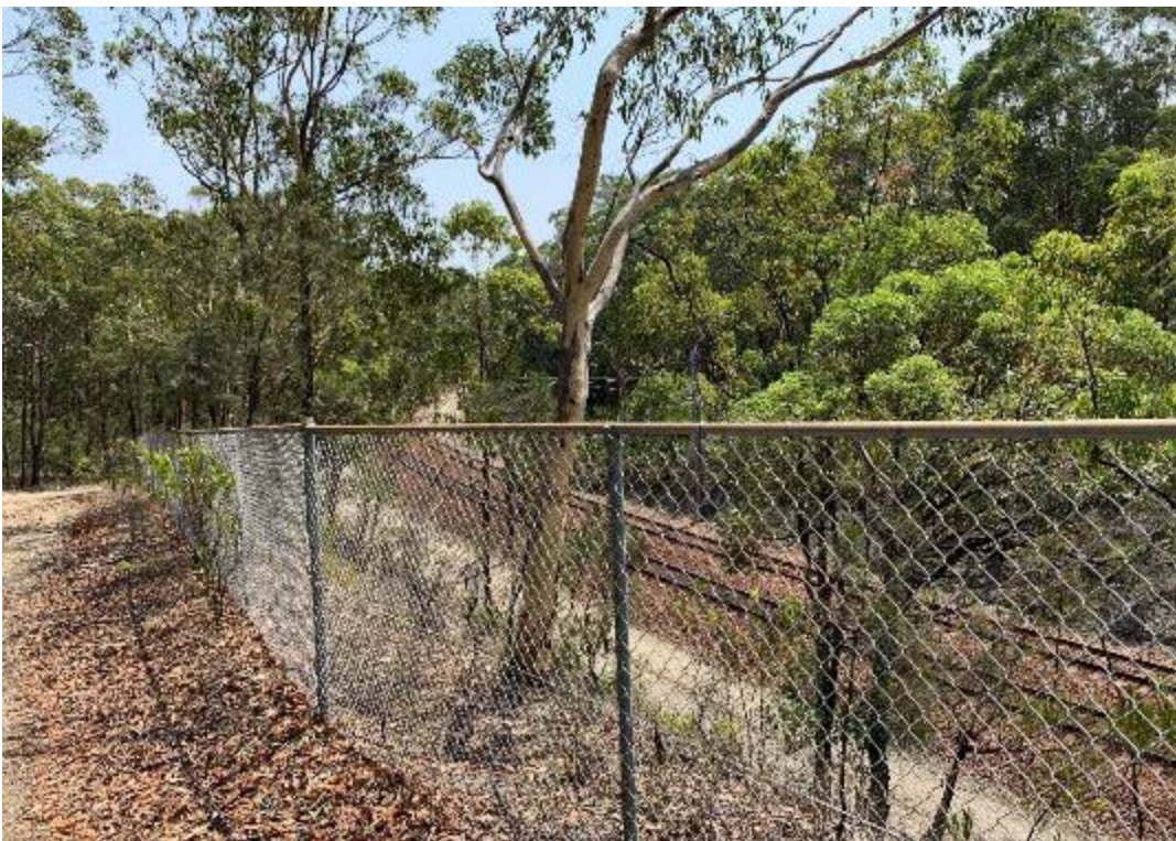
Plate 5.4 View of the Main Northern Railway, in proximity to the northern boundary of the Extension of Mining Area
