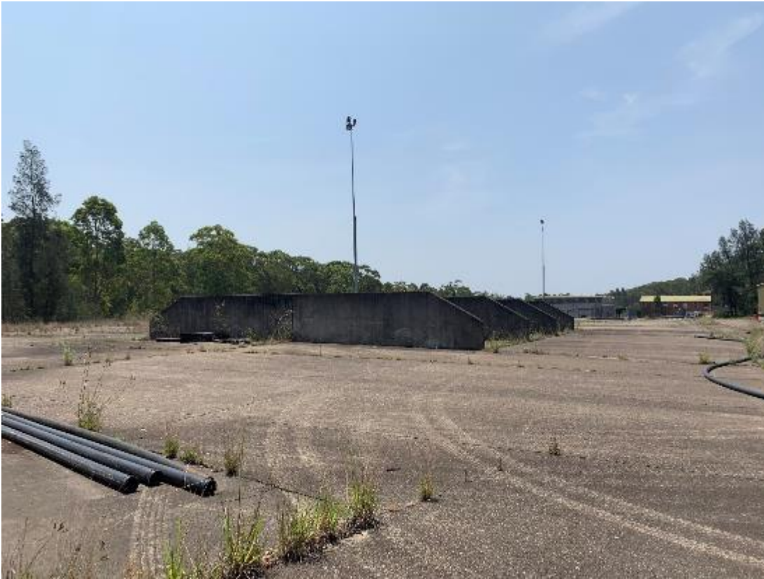
Plate 5.11 The concrete material storage areas will be removed as part of the current proposal. These are not identified as significant in the 2012 RPS report.
