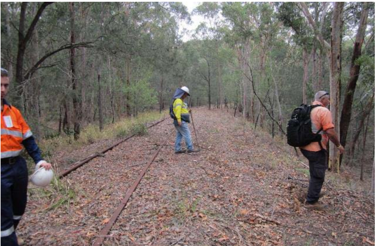
Plate 5.17 View of a section of the Line that extends along an embankment
