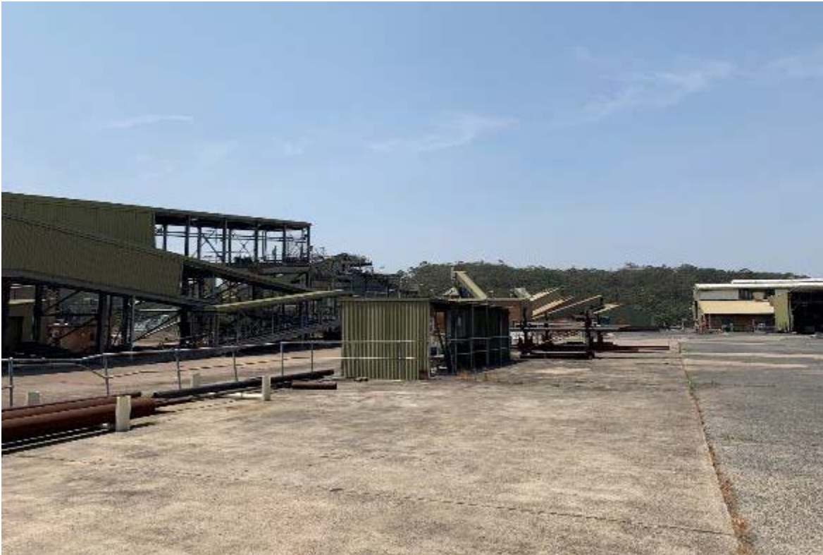
Plate 5.6 Views within Newstan Colliery, showing post-1948 building stock
