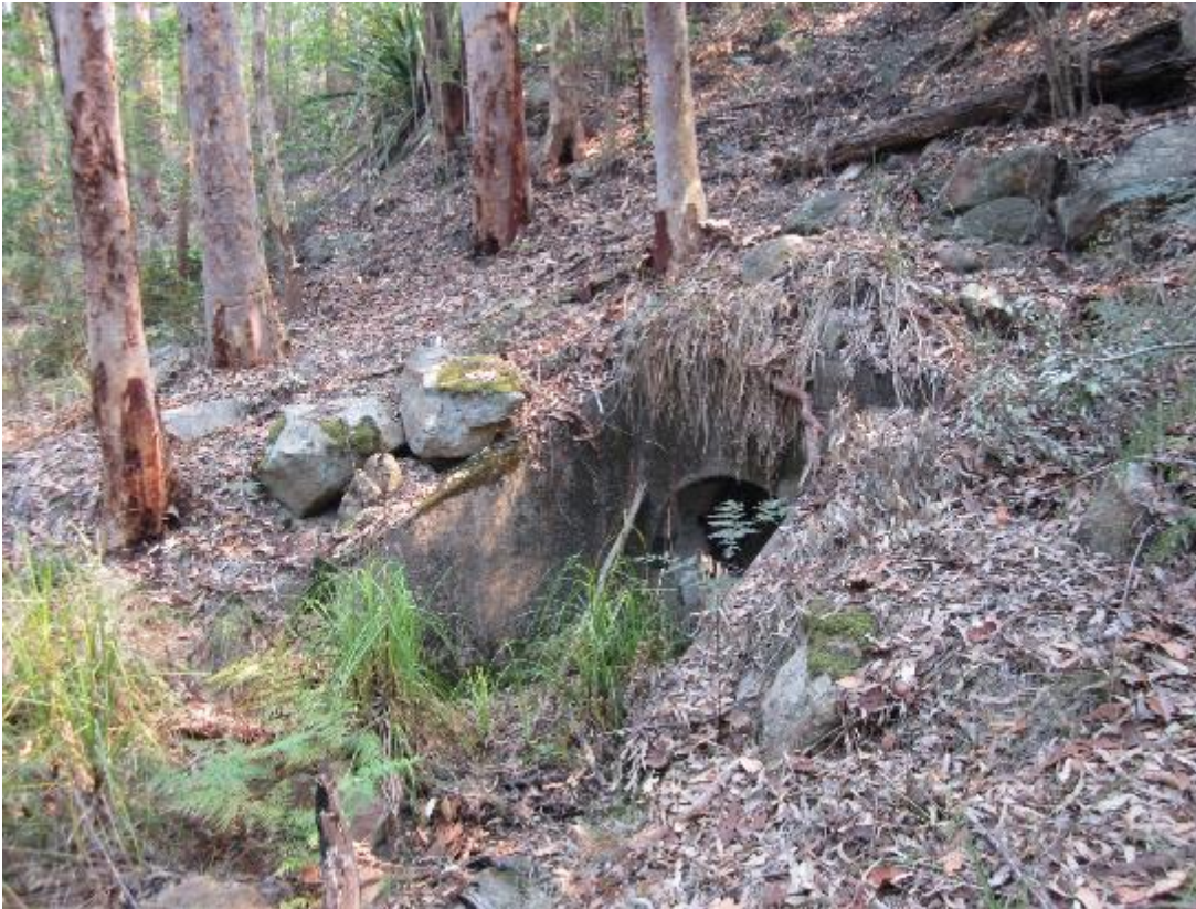
Plate 5.18 Example of a culvert within an embankment along which the Line extends
