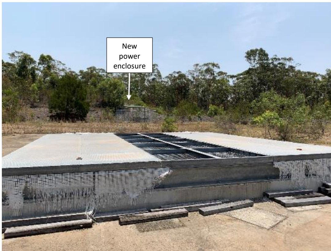
Plate 5.8 Existing ventilation shaft. A fan house is to be built over the shaft. A new power enclosure will be constructed as indicated.
