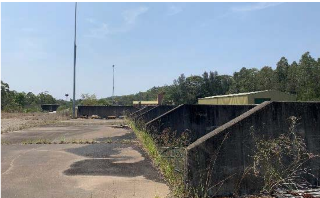
Plate 5.12 The concrete material storage areas will be removed as part of the current proposal. These are not identified as significant in the 2012 RPS report.
