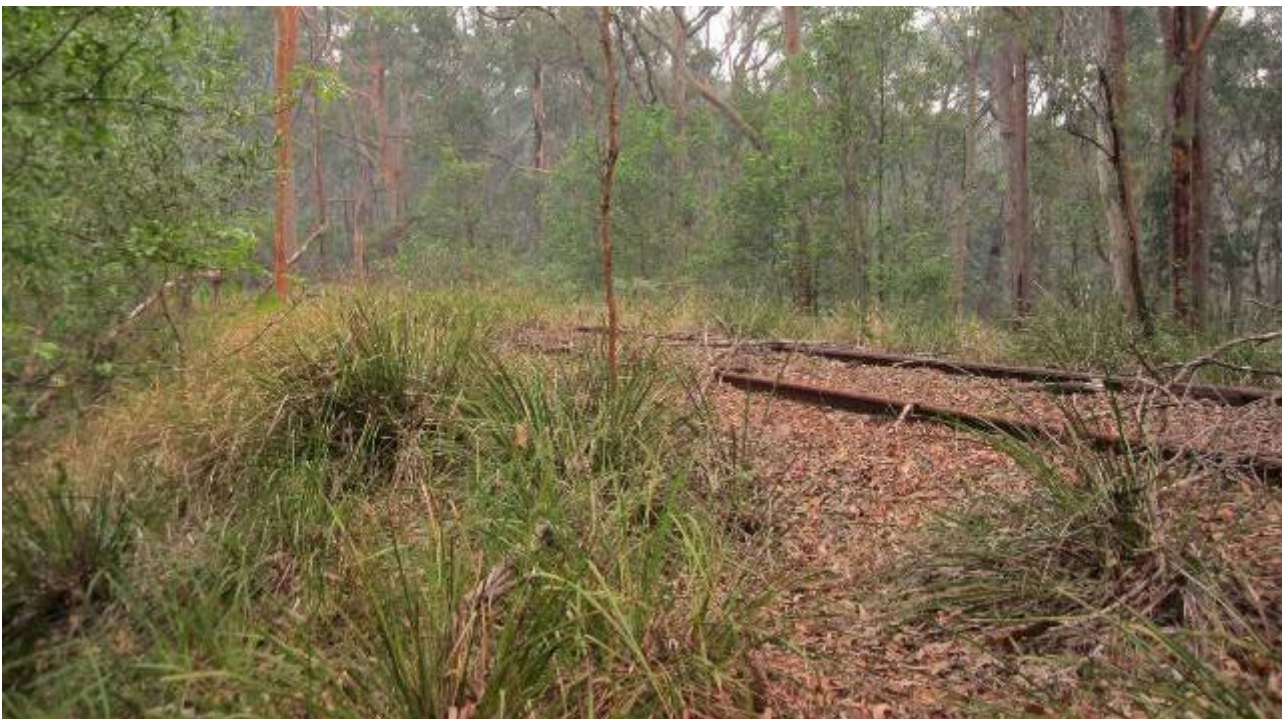
Plate 5.19 View of a section of the Line that extends along an embankment
