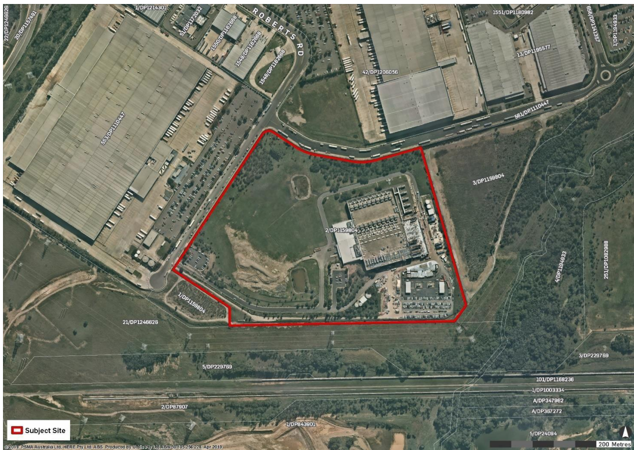
Figure 1 Aerial imagery of the Site
