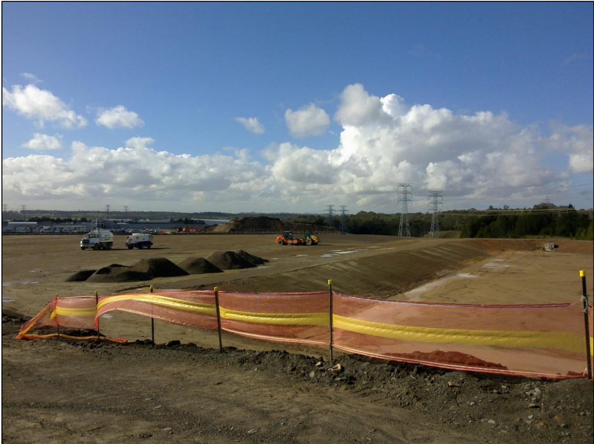
Figure 7: Pit 2 area in June 2011 after completion of backfilling
