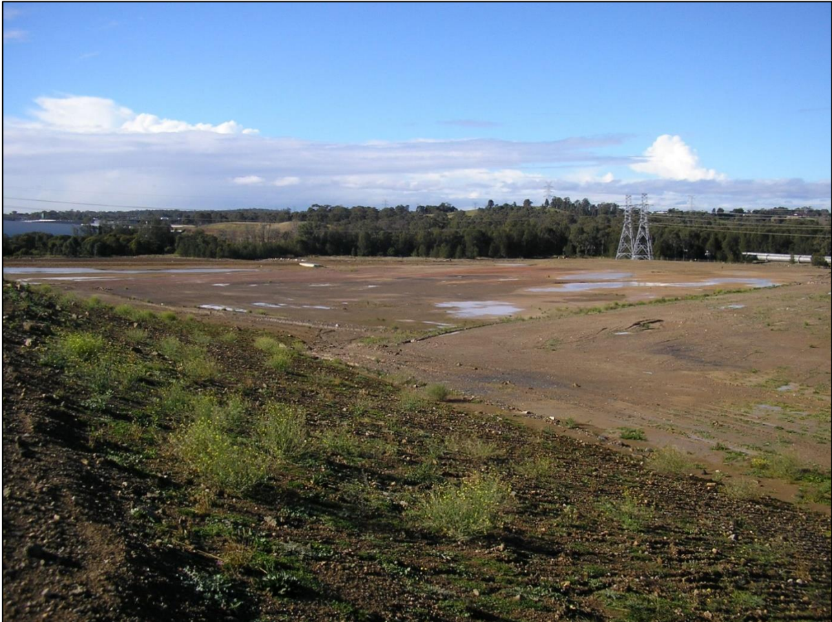
Figure 4: View of Pit 1 after completion of back filling – looking south east
