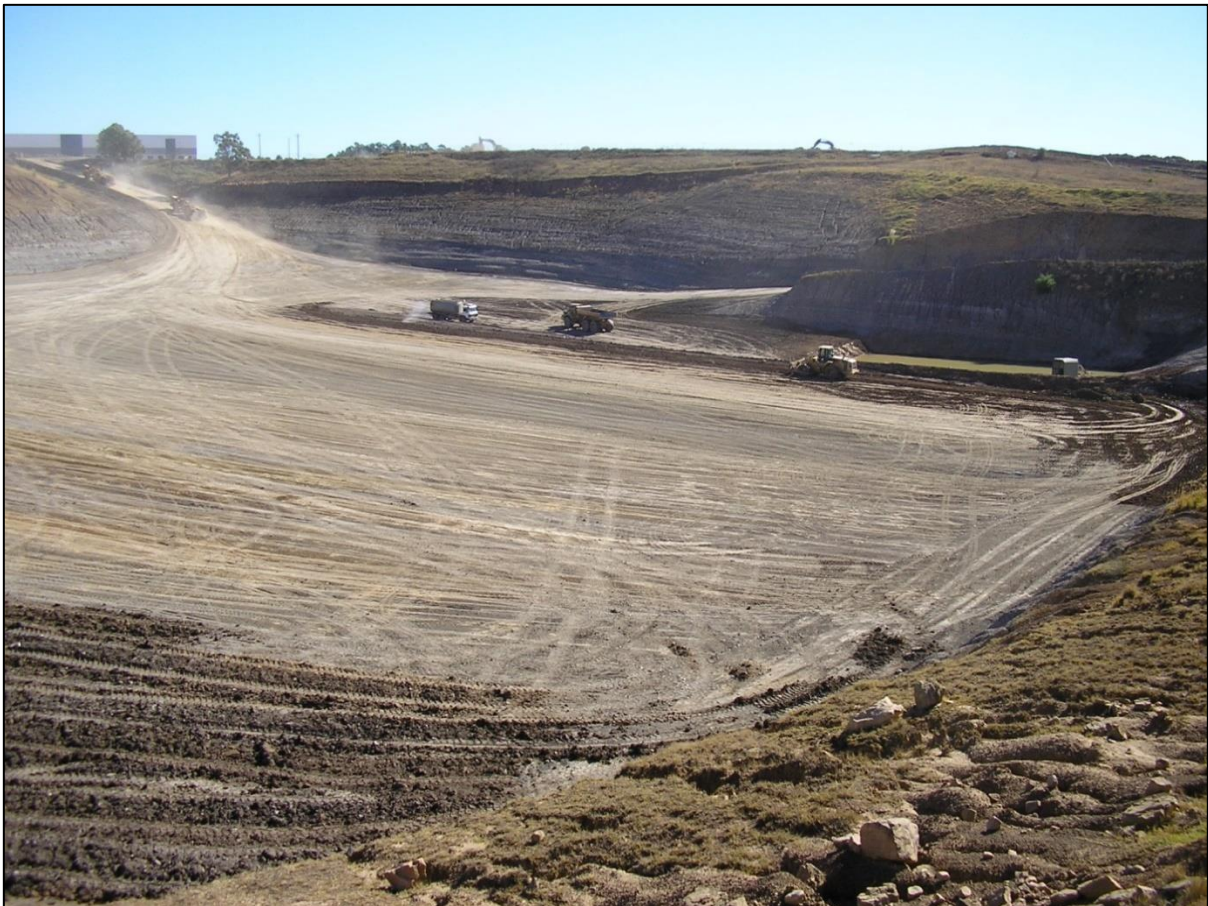
Figure 3: Backfilling of Pit 1 in May 2006
