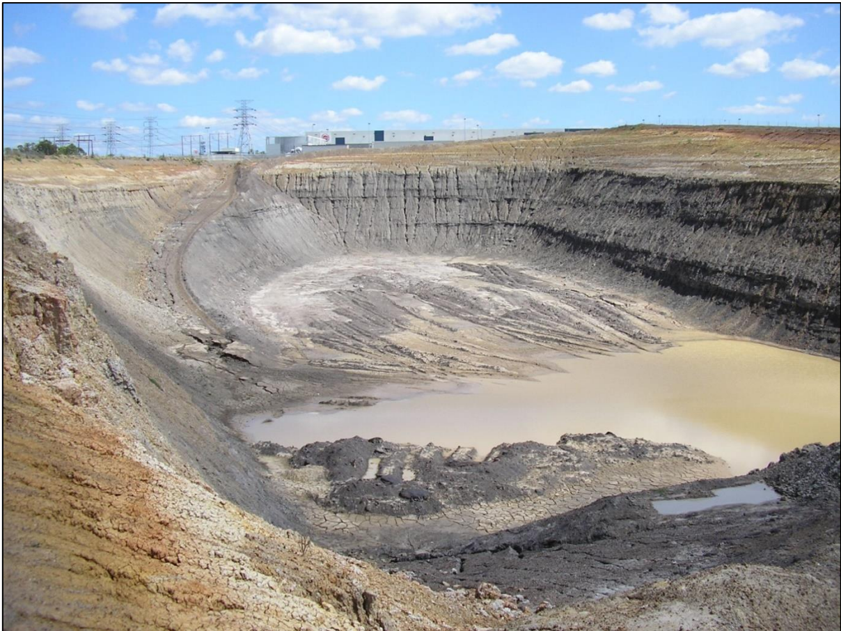
Figure 5: View of Pit 2 in October 2008 prior to backfilling
