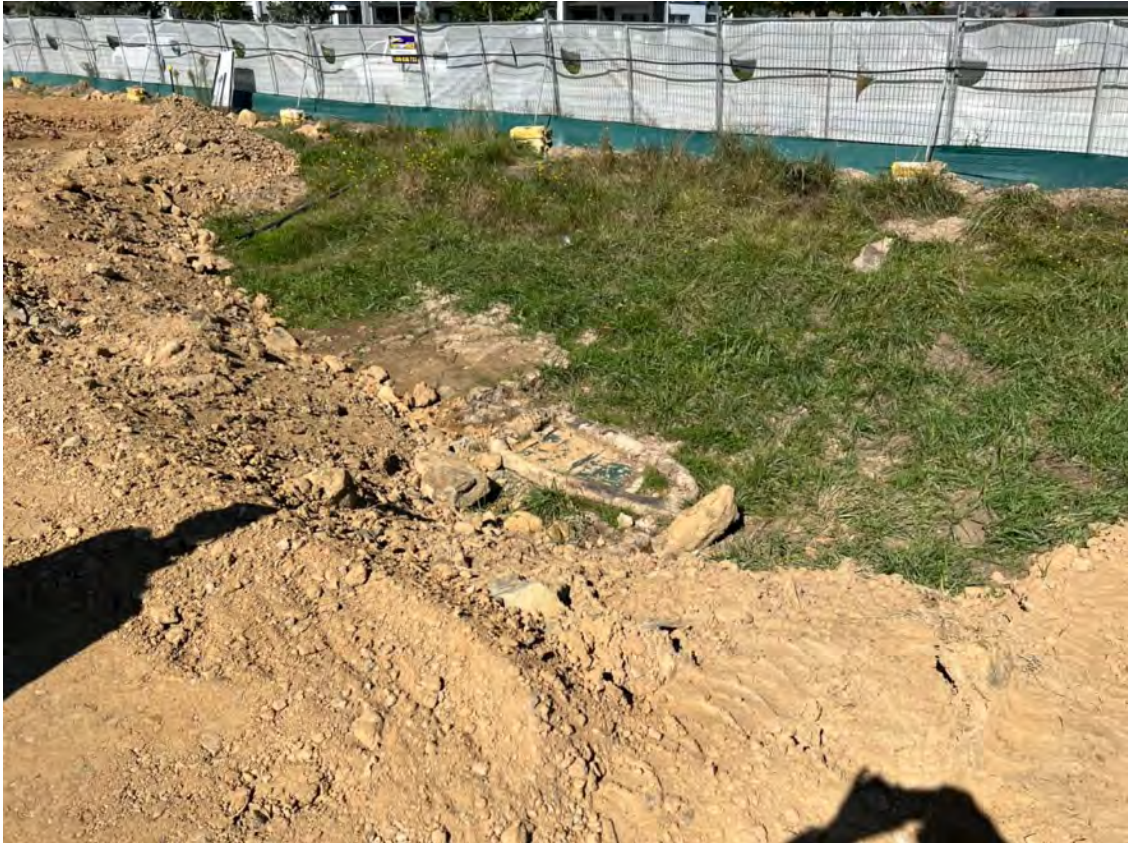
Photo 5 Blocked stormwater drain requires maintenance
