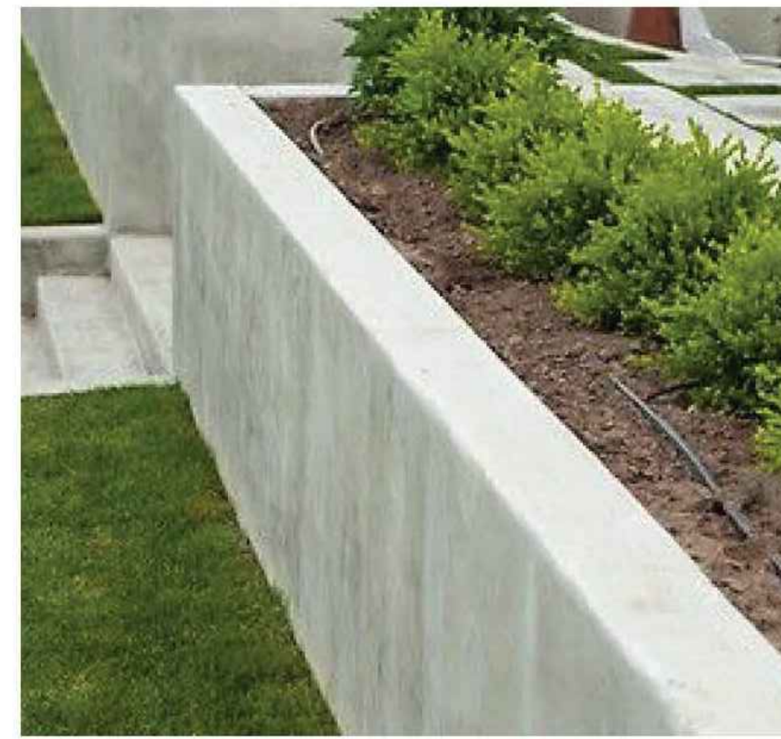
In-situ concrete walls
