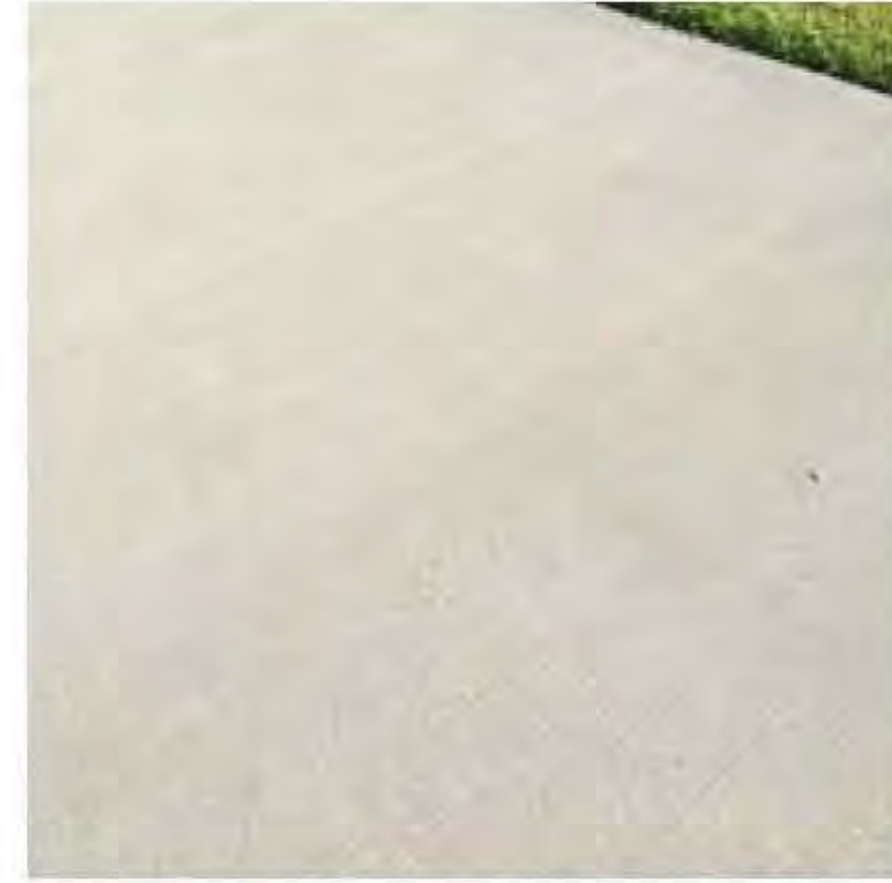
Concrete - Oxide finishes
