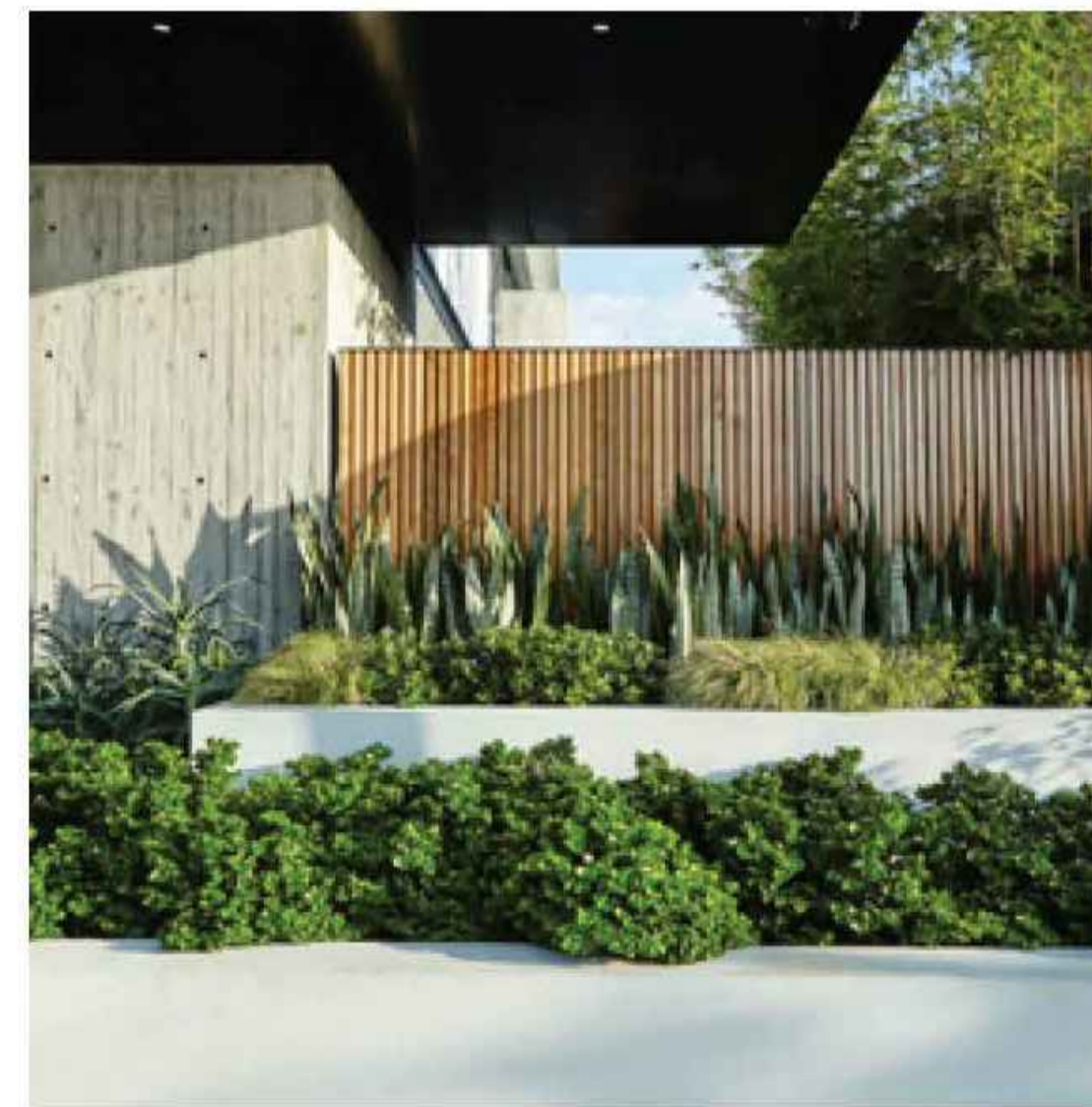
In-situ concrete planter box
