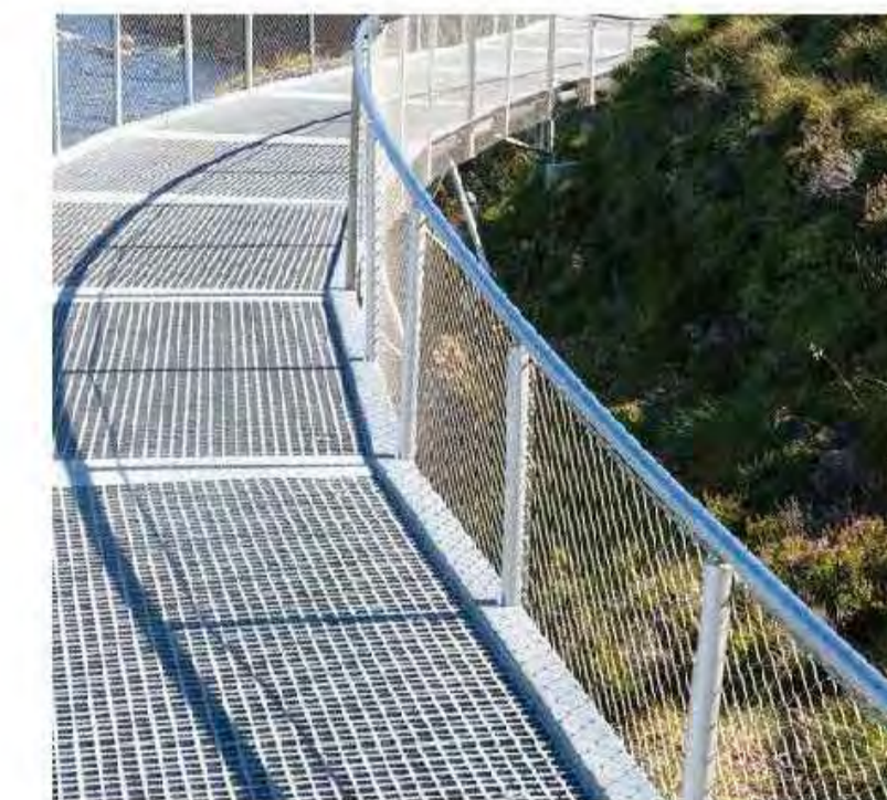
Aluminium boardwalk structure
