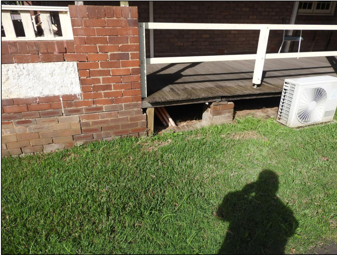
Figure 5.14 Foundations of house including visibility of underneath soil exposure. Facing west, (AMAC 2020, Photo No. DSCN3935).
