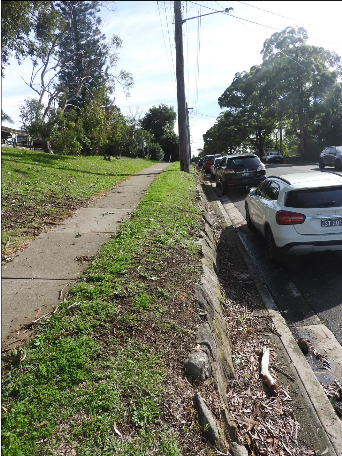
Figure 5.18 Eastern boundary of study area. Illustrating sandstone wall retaining roadside fill level above road height. Facing north, (AMAC 2020, Photo No. DSCN3929).
