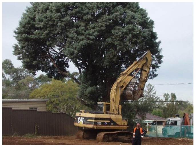
Photo 12: Keep equipment away from the tree by using appropriate tree protection.
