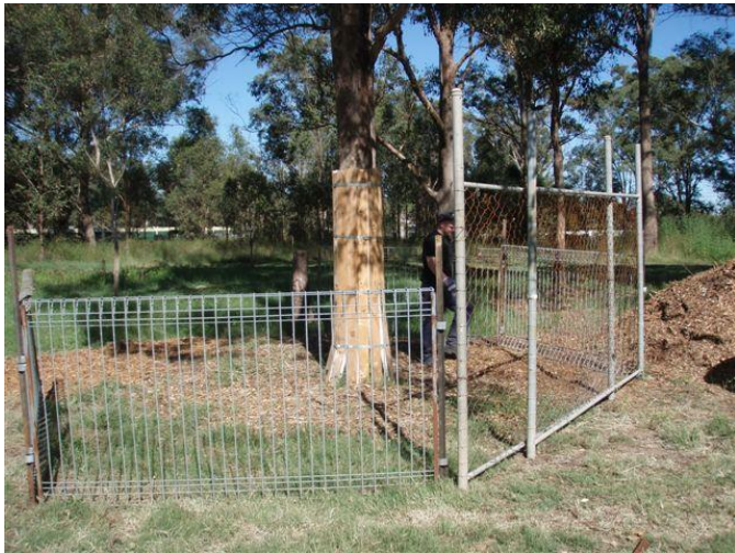
Photo 1: The fence should be rigid and hard to move.
