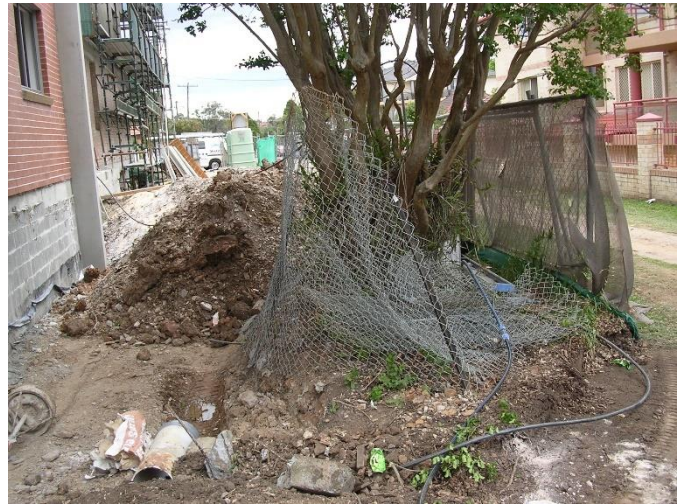
Photo 2: This style of fence is too easily damaged and collapses when hit.
