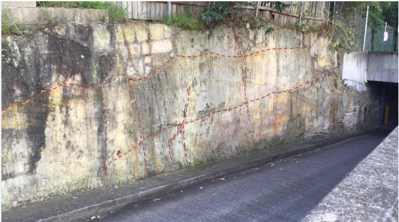
Plate 2 - Rock exposure, containing defects, along the northern site boundary – Looking towards the west
