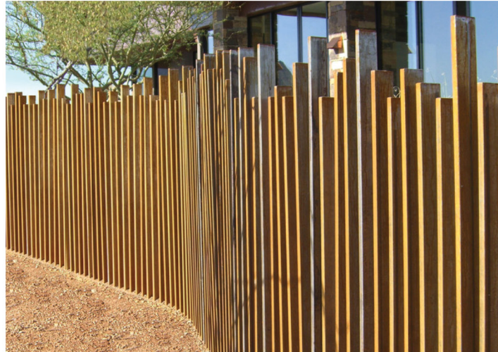
FENCE TYPE B - STEEL SLAT FENCE
