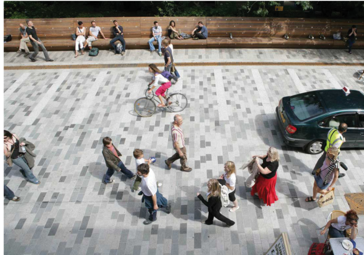
PAVING TYPE 1 - CONCRETE UNIT PAVERS, GREY TONES
