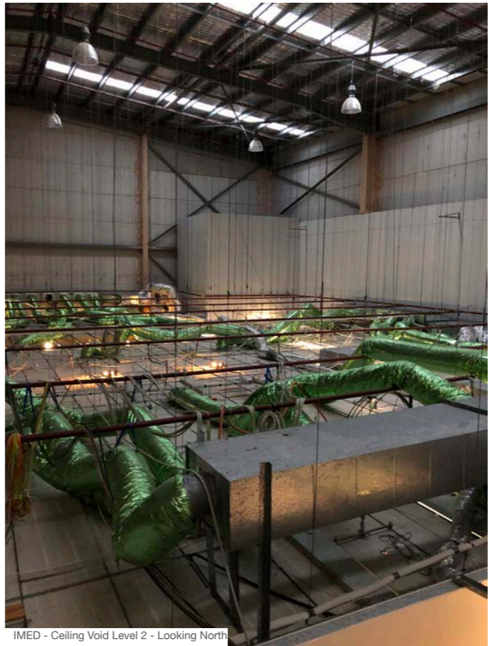
IMED - Ceiling Void Level 2 - Looking North
