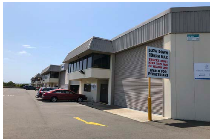
View 19 - Looking north along western facade of 224 Headland Road. Source: TZG Architects, 2019
