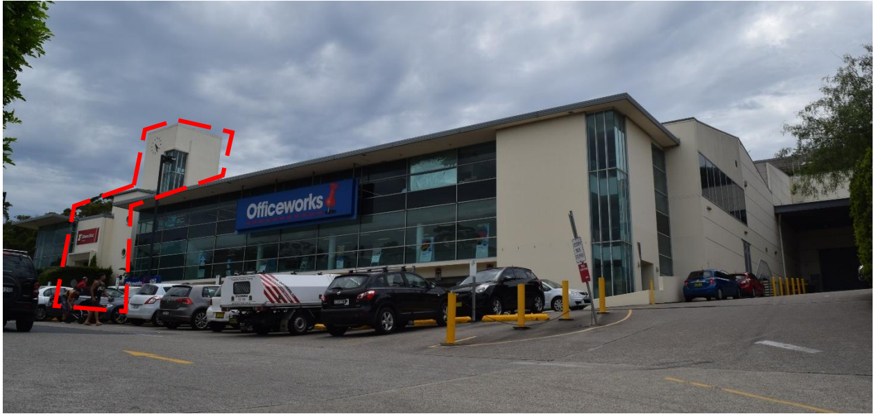
Figure 33: Looking northeast toward the western façade of the subject building within 800 Pittwater Road, from the south-west corner of the site. Note: The area identified as heritage fabric is indicated in red. Original fabric (building footprint) along the western elevation includes the structure below the glazing.
