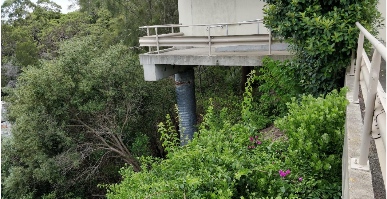
Figure 59: The remainder of the building is supported on columns above a densely-vegetated and steep section of the hillside (Source: TZG Architects, May 2019).
