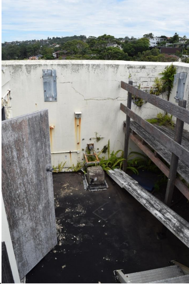
Figure 49: Image showing the condition of the roof-top of the clocktower including wooden platform and surface mounted conduits.
