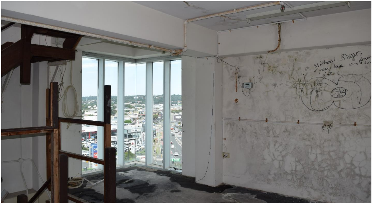
Figure 48: Looking towards the top-floor window within the clocktower. Note: Interior graffiti to the internal walls and rising/falling damp.
