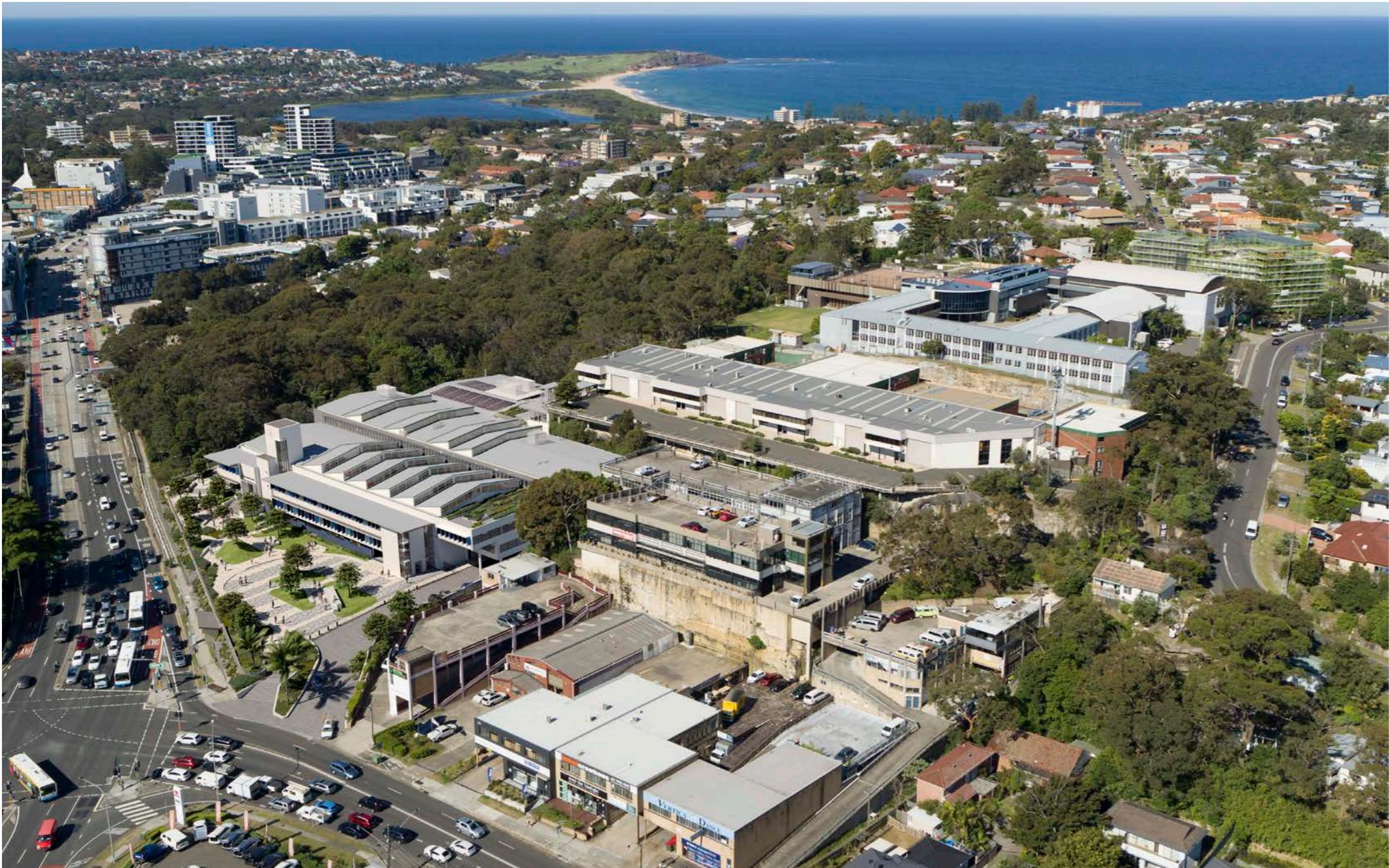
View from Pittwater Road
