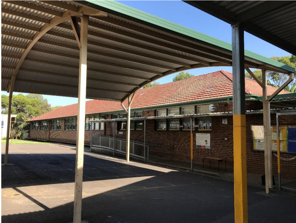
Figure 39 Southern Elevation of Block I (former Infants Building) (January 2019)
