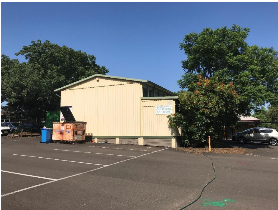
Figure 38 Block K is a fibre cement clad modular building. It currently houses storage from the NSW Schools Sports Unit (January 2019)
