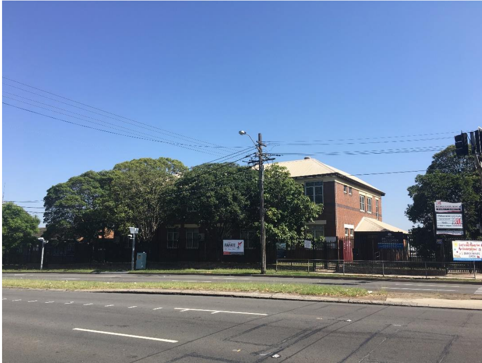
Figure 26 View of Block A from the southern side of Hume Highway (January 2019)
