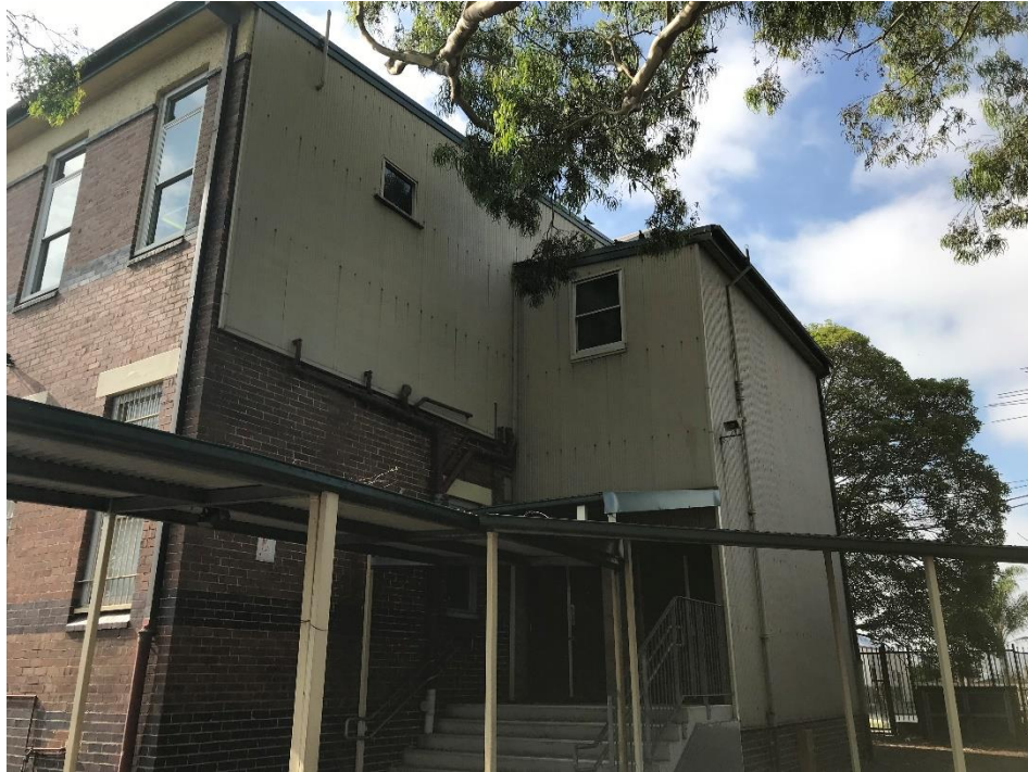
Figure 24 Western Elevation with metal sheet clad staircase (January 2019)
