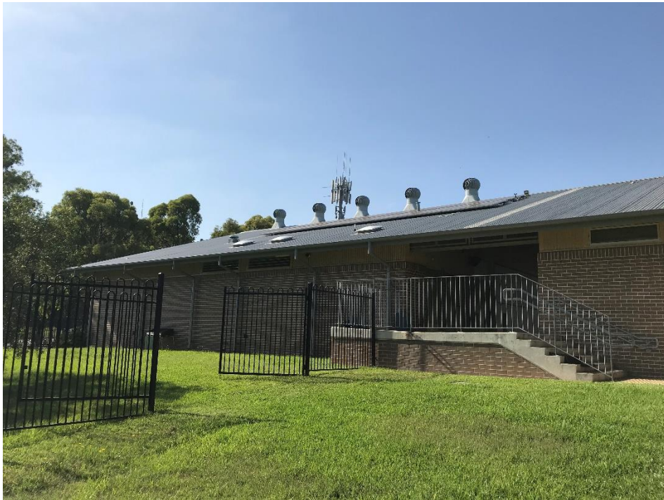
Figure 40 Block N (hall and canteen) dates from 2010 and was constructed as part of the Australian Government's Building Education Revolution funding programme (January 2019)
