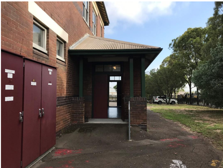
Figure 23 Entry Porch (January 2019)
