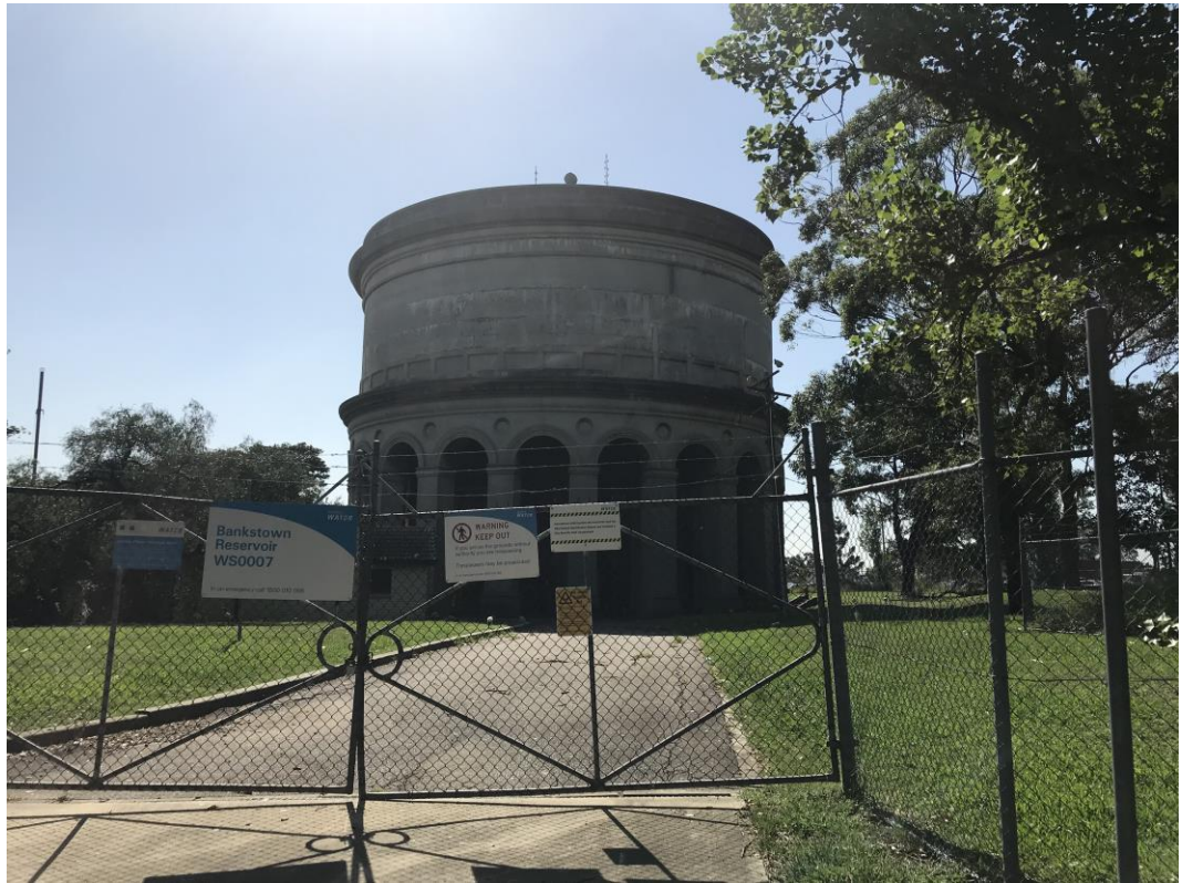
Figure 44 Bankstown Reservoir as viewed from Beresford Avenue (January 2019)
