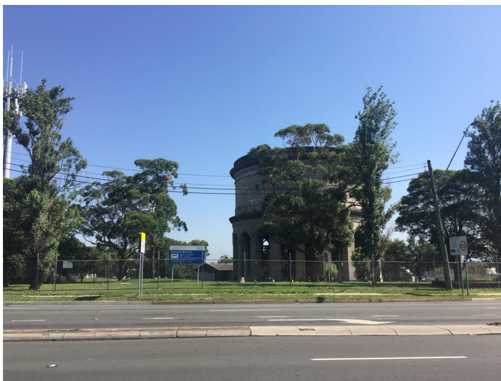
Figure 52 Bankstown Reservoir (Elevated) as viewed from the south side of the Hume Highway (January 2019)
