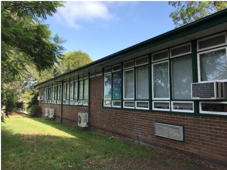
Figure 34 Southern Elevation of Block B (January 2019)
