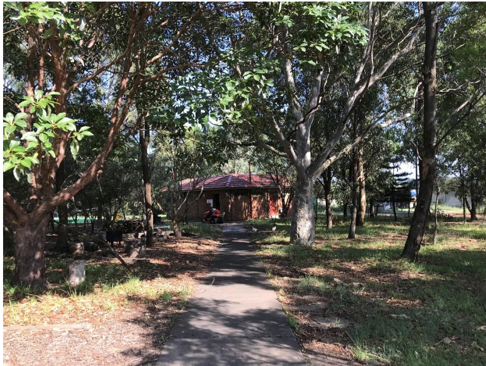
Figure 41 Block J is currently used for storage (January 2019)
