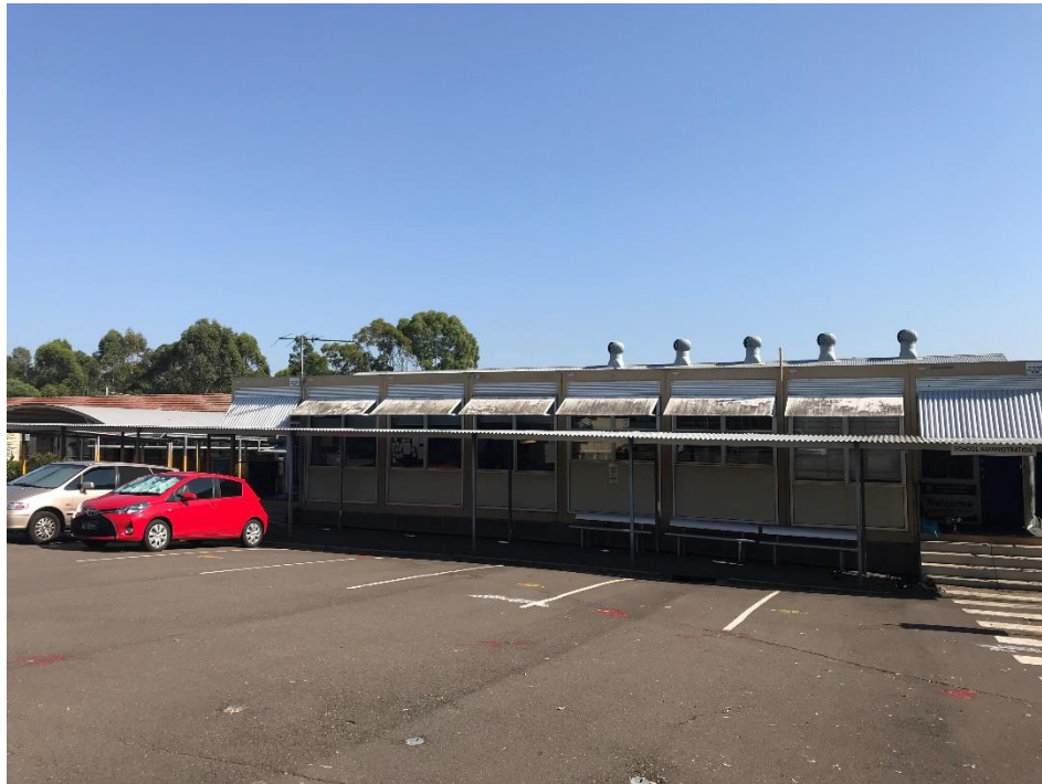
Figure 43 Administration block (dismountable) (January 2019)
