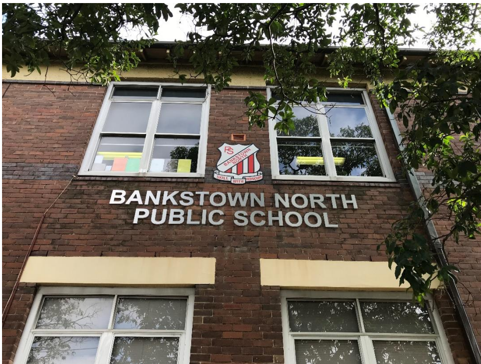
Figure 27 The old sign identifying the name of the school and year of construction has been removed (visible in the 1924 image) and replaced with modern signage (January 2019)
