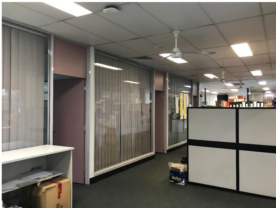
Figure 32 The first-floor assembly hall has been converted for use as an office space with lightweight partitions and suspended ceiling tiles (January 2019)
