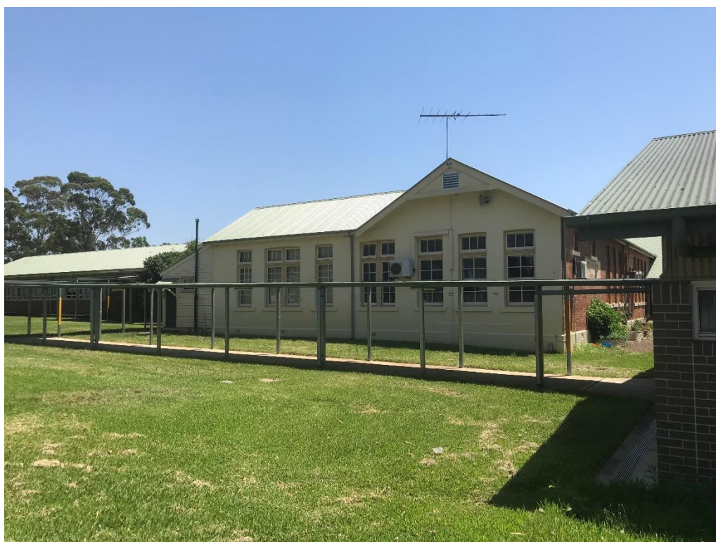
Figure 51 Revesby Public School (January 2019)
