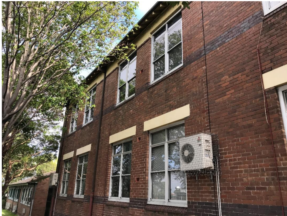
Figure 25 Southern elevation of Block A with aluminium double hung windows. The junction between the 1924 building and the 1928 extension is clearly visible. The elevation has been kept relatively uncluttered by air conditioning units (January 2019)
