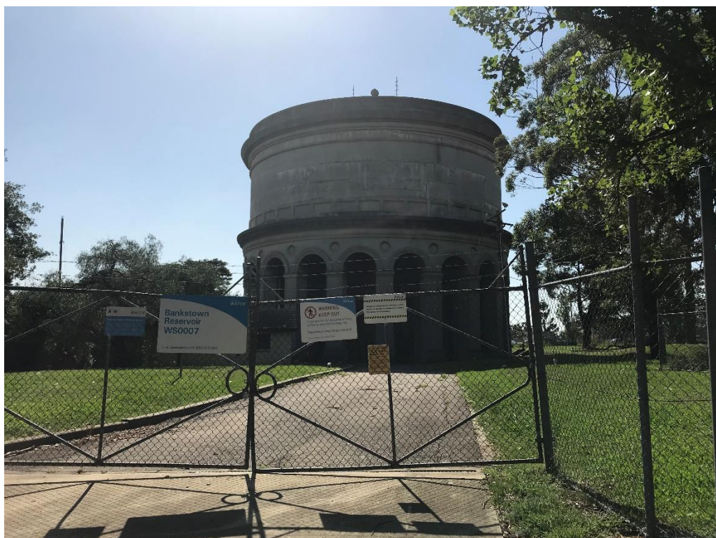
Figure 12 Bankstown Reservoir (Elevated) as viewed from Beresford Avenue (January 2019)
