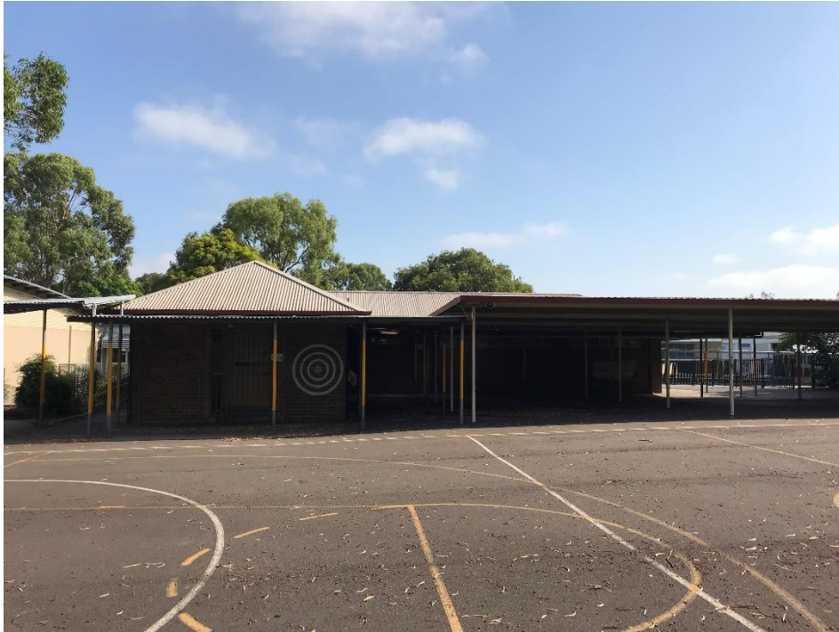
Figure 35 C Block with associated COLA (January 2019)
