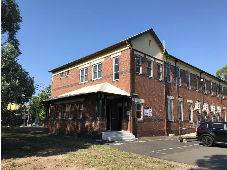
Figure 22 Eastern Elevation of Block A (January 2019)
