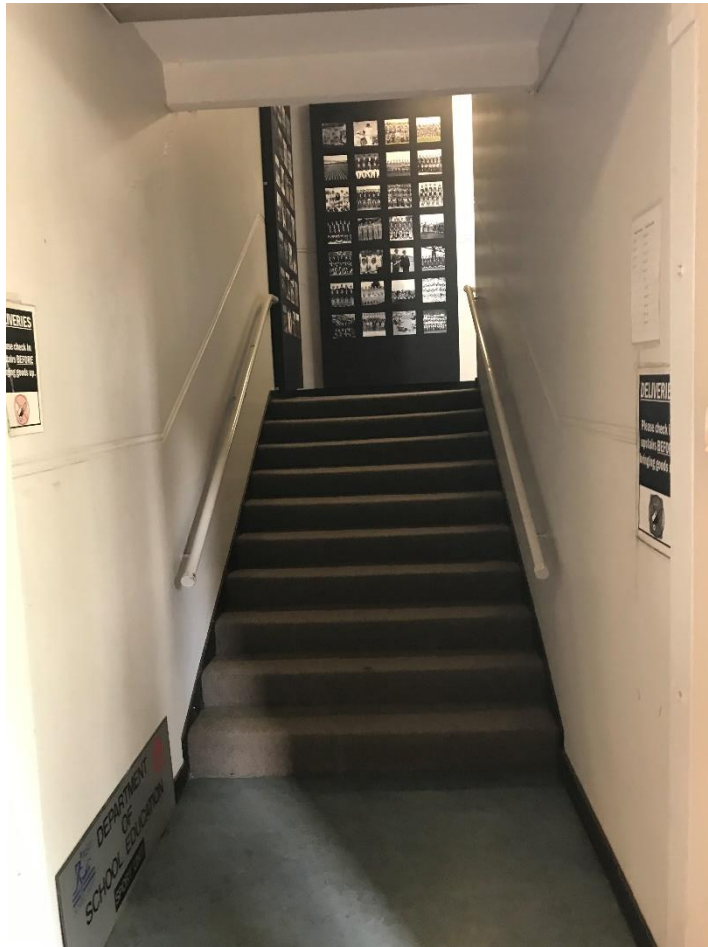
Figure 31 Stairs to the first floor (January 2019)
