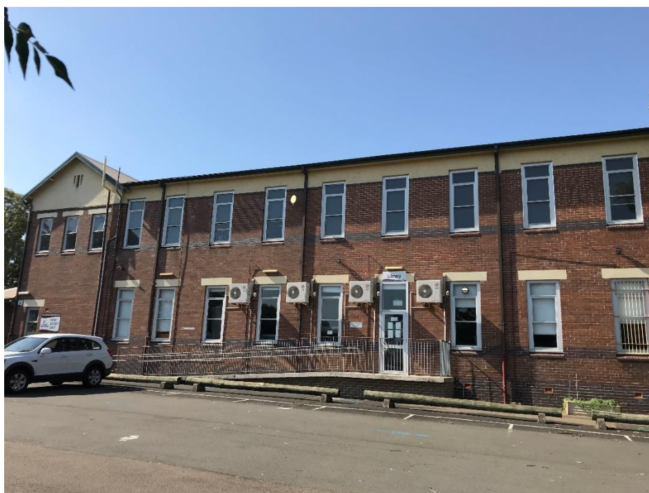
Figure 28 Northern elevation of Block A (January 2019)
