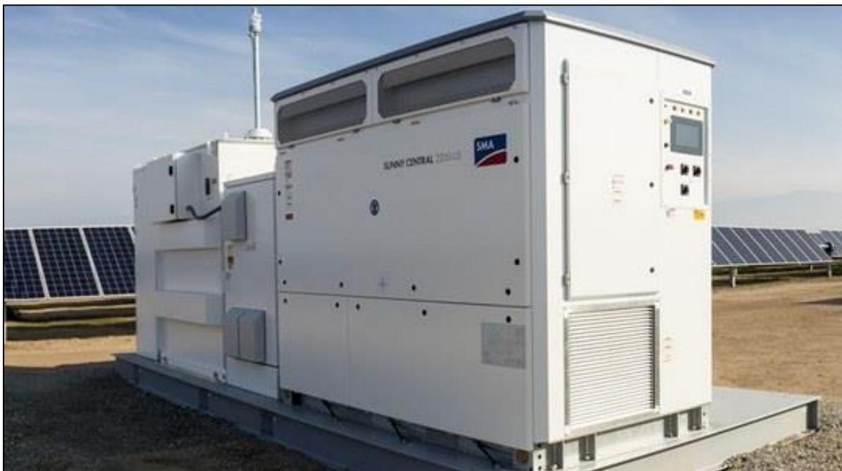
Figure 3-15 Containerised inverter/transformer unit with battery storage.
