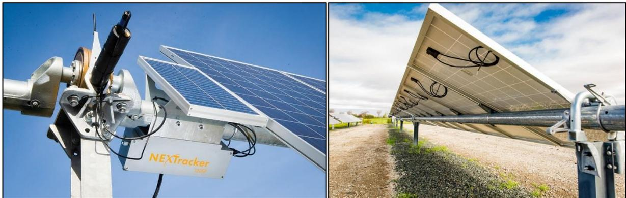
Figure 3-13 NexTracker single axis tracking system.
