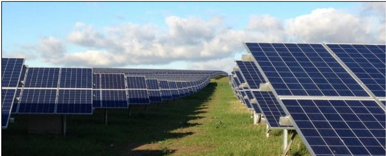
Figure 3-11 Example of 2 m x 1 m solar panels arranged in rows.
