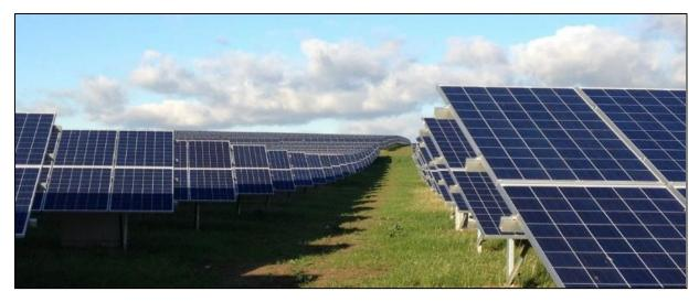
Figure 3-11 Example of 2 m x 1 m solar panels arranged in rows.
