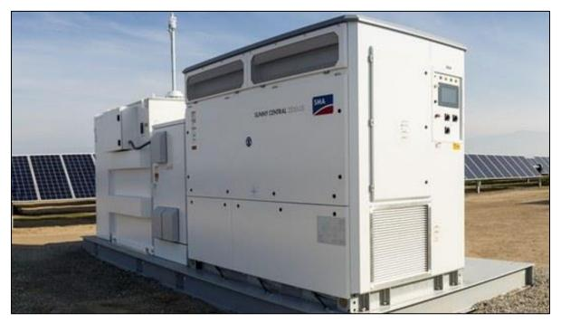
Figure 3-15 Containerised inverter/transformer unit with battery storage.
