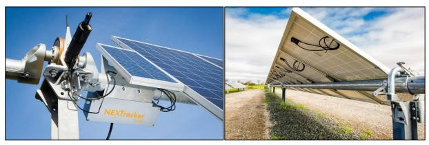
Figure 3-13 NexTracker single axis tracking system.
