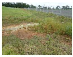
Figure 9 – Erosion exposure within embankment between hardstands. Aspect south
