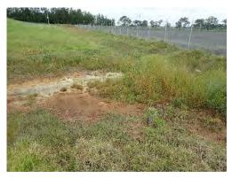
Figure 27 – Erosion exposure within embankment between hardstands. Aspect south
