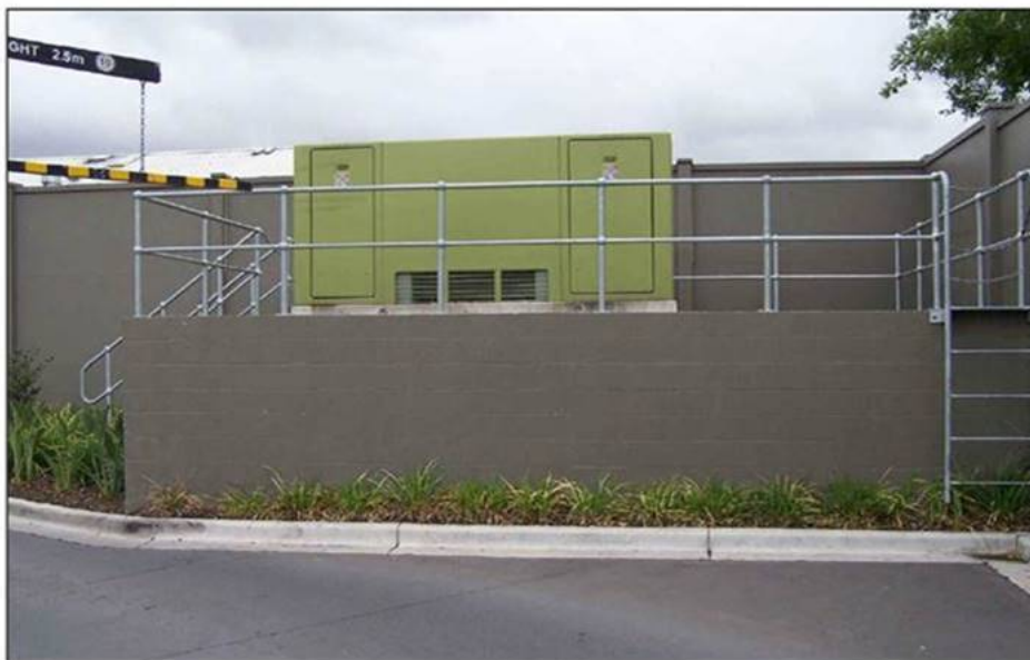
Figure 51 - Example substation raised above 1:100 flood level
