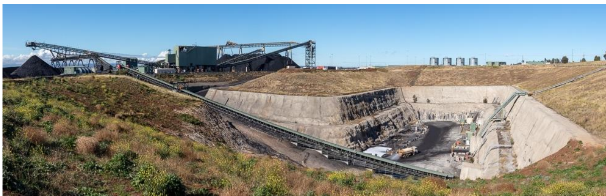
Plate 2-1 Narrabri Mine Box Cut and Drifts
