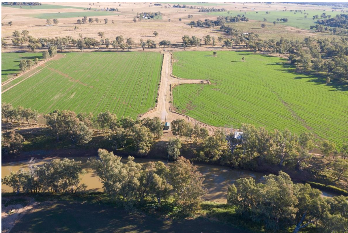
Plate 2-5 Existing Namoi River Pump Station and Production Bore
